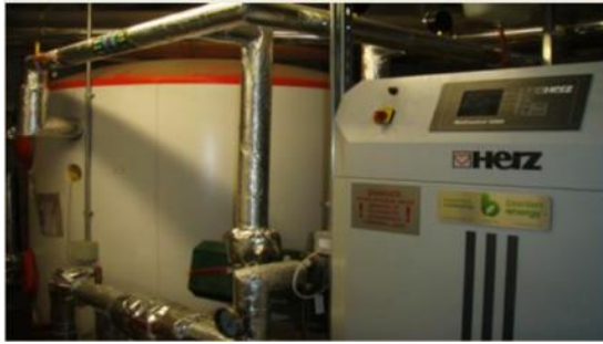
Figure 4-61. Biomass boiler
