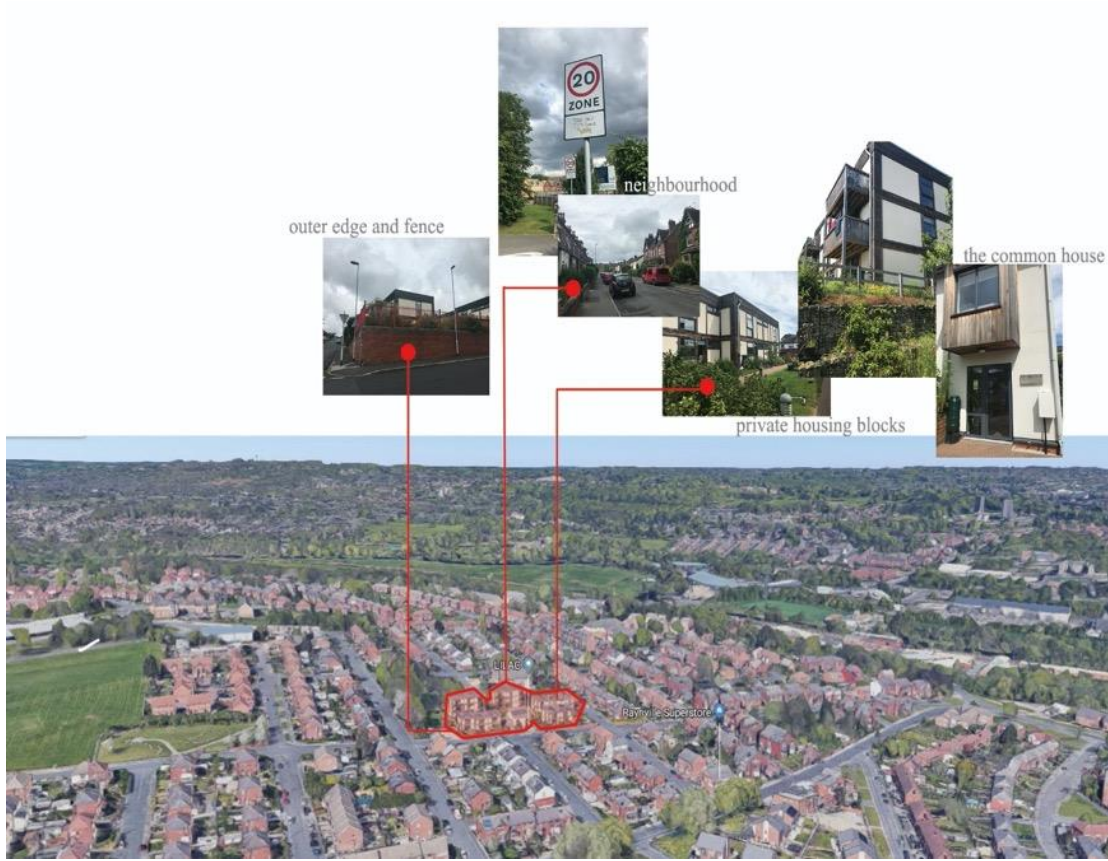
Figure 4-3. Site location and surrounding neighbourhood
