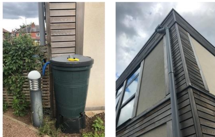
Figure 4-22. Rainwater collection system
