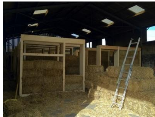
Figure 4-18. Panel timber and straw-bale Source: LILAC
