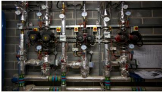
Figure 4-62. District heating controls
