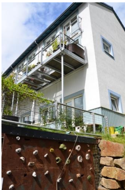
Figure 4-74. The climbing wall
