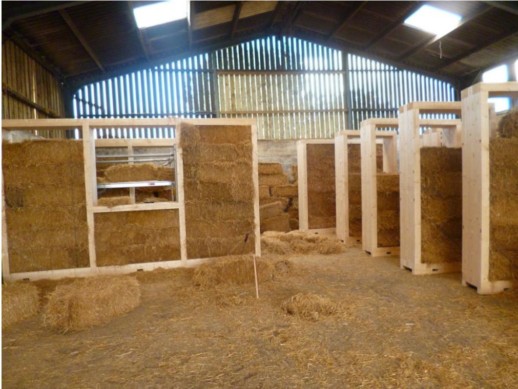
Figure 4-19. Timber frame and straw-bale. Source: LILAC
