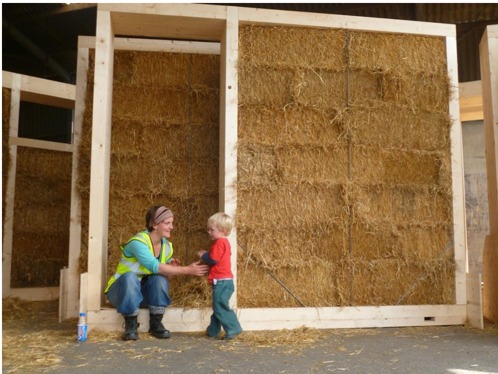
Figure 4-20. cohousing residents and children involved in the straw-bale construction process. Source: LILAC
