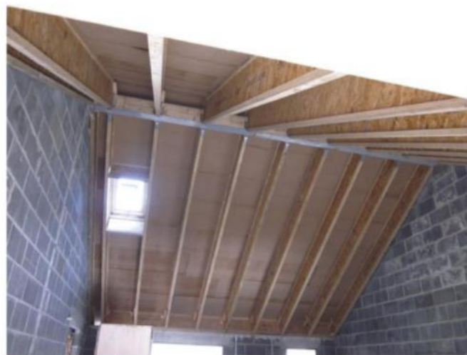
Figure 4-60. ceiling structure (Eco arc)
