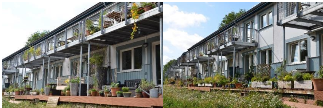
Figure 4-70. Front side of the terrace
