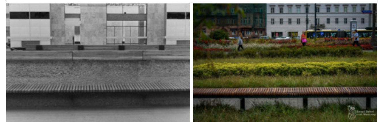
ill. 9.42 and 9.43 - interior of Warsaw Midtown railway station in the 1960s and today, showing remaining elements from the initial concept (travertine wall cladding, concrete floor cladding and hanging sound insulating rack; throughout the years although the cladding of the columns was changed, and the illumination was replaced with one hanging below and not above the rack (making it impossible to illuminate the ceiling and to expand the space visually as it was intended initially); in addition, the track ditch has now become a black line cutting through the interior, something that was avoided in the design
