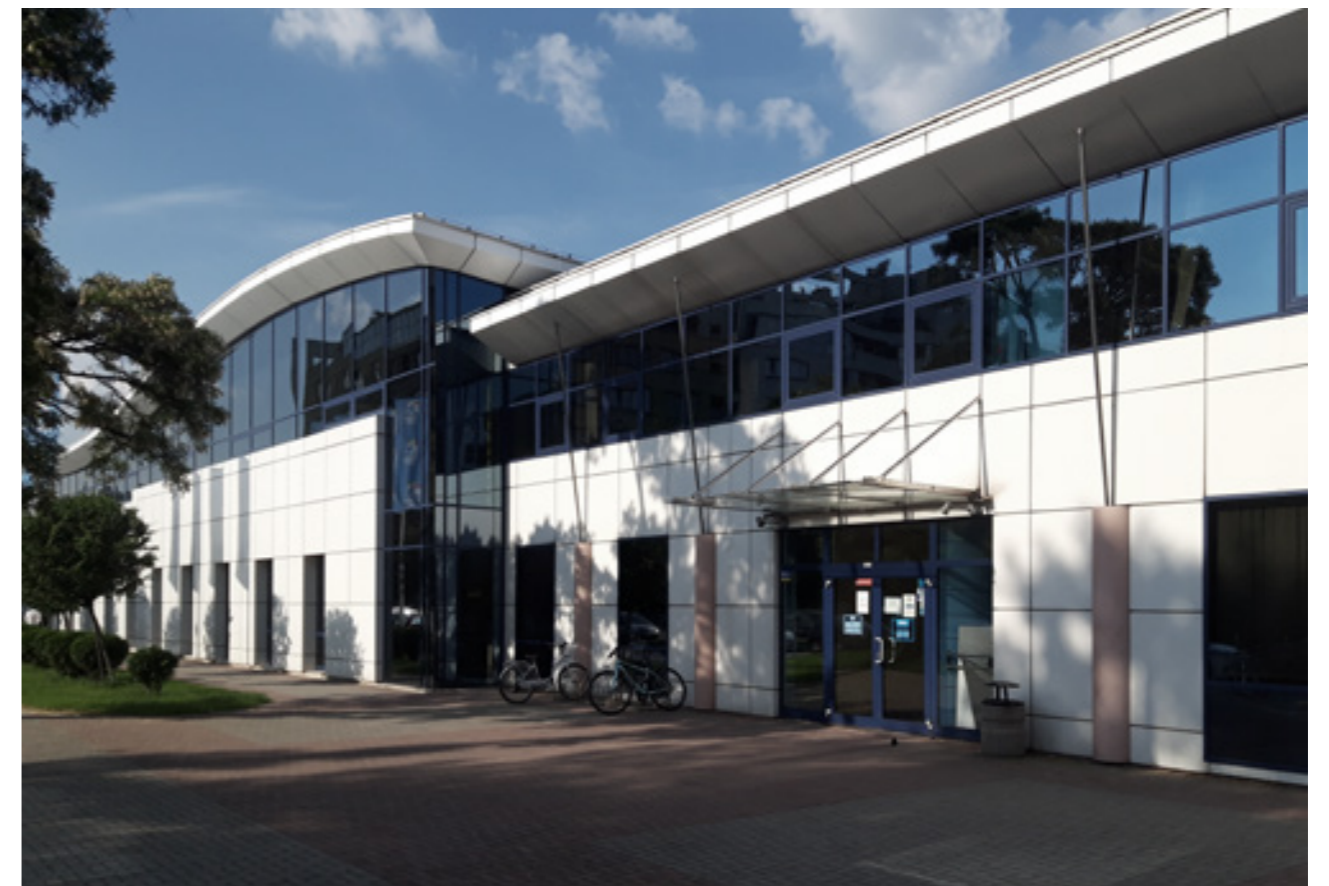
ill. 9.30 – closed pavilions at the centre of the main stadium as an example of incompatible modifications within the site
