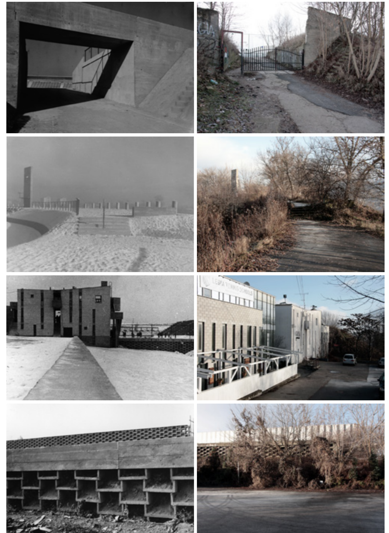
ill. 9.22, 9.23, 9.24, 9.25, 9.26, 9.27, 9.28, and 9.29 - comparison of ‘Warszawianka’ sporting centre when it was fully operative (1970s) and its present-day state in different parts of the complex, pointing to the severe issues linked to the lack of maintenance since its opening; the main stadium and the connection to the lowest terrace (top line) show particular signs of negligence, whereas the circular path around the main stadium (second line) has become unrecognisable underneath shrubberies; the office pavilion next to the tennis/hockey stadium (third line) and the retaining walls (bottom line) are best preserved thanks to the maintenance works from the early 1990s
