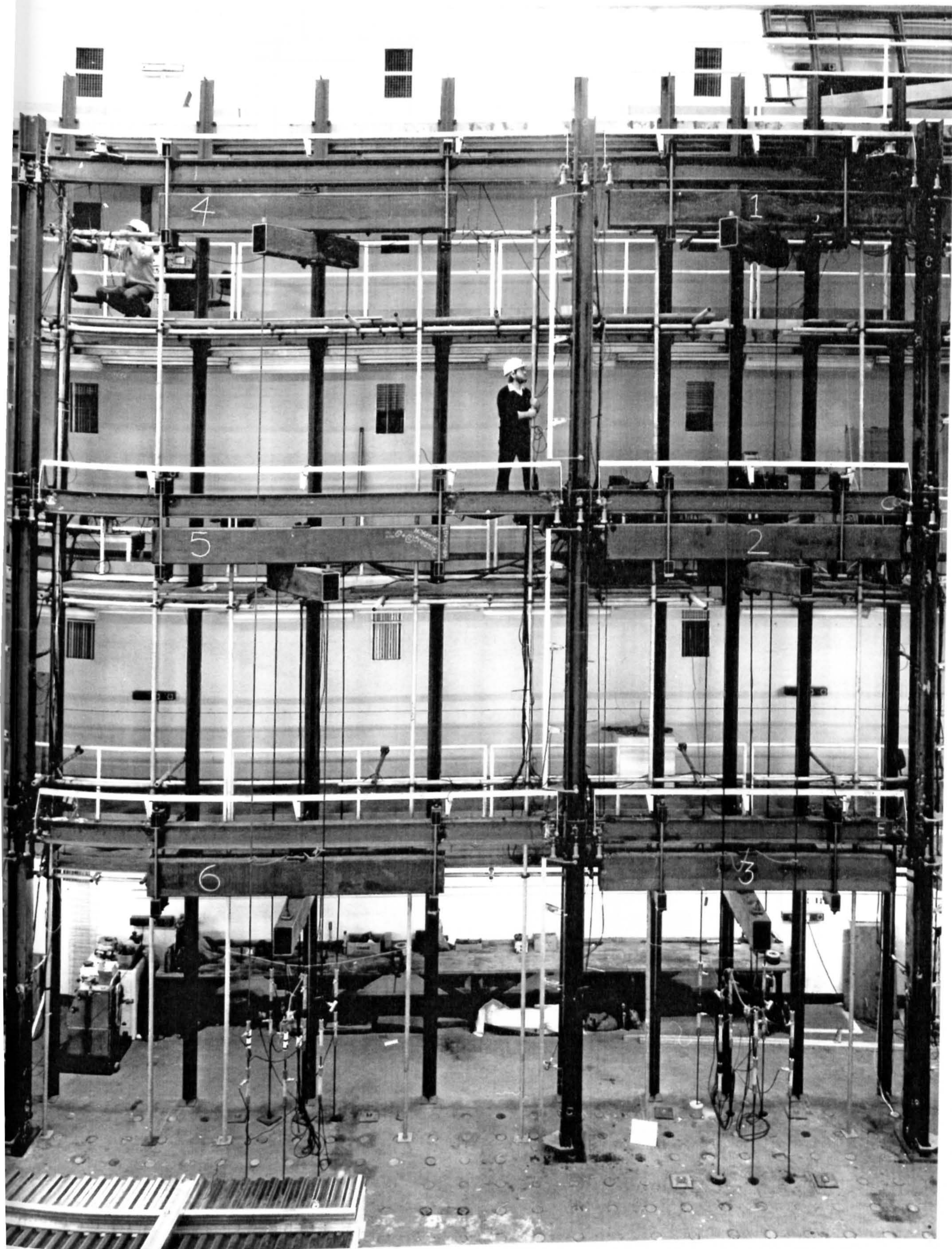
Figure 5.1 : Frame 1 viewed towards the Balcony
