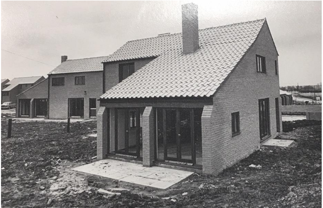
Fig.24. House on Kindleton in Great Linford. 1978. Photographer: Bilton Studios for the Milton Keynes Development Corporation. D-MKDC/16/1/9. Centre for Buckinghamshire Studies.
