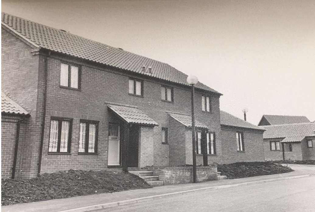
Fig.41. Rental houses in Nicholas Mead, Great Linford. Taken February 1980 by Ivor Leonard for the Milton Keynes Development Corporation. D-MKDC/16/1/9. Centre for Buckinghamshire Studies.
