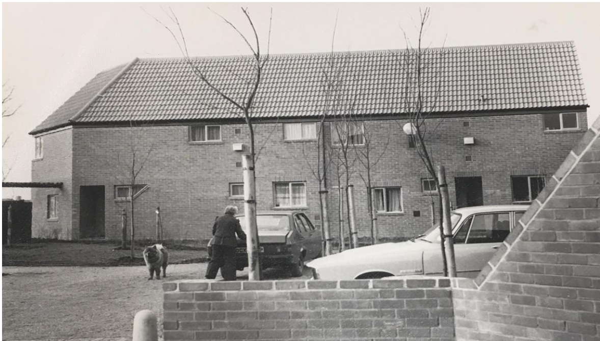
Fig.36. View of rental houses from adjacent parking. France Furlough in Great Linford. Taken 10 January 1980 by Ivor Leonard for the Milton Keynes Development Corporation. D-MKDC/16/1/9. Centre for Buckinghamshire Studies.
