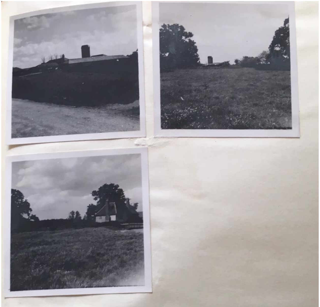
Fig.17. 1946 journal entry with photographs of the site that would become Harlow New Town. FG1/29. Gibberd Garden Archive.
