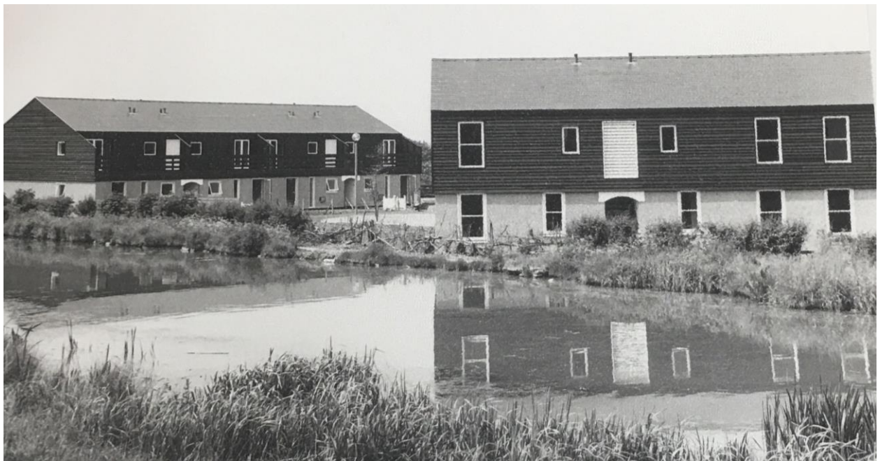
Fig.38. Great Linford's "Campion" rental houses. Taken by Bilton Studios for the Milton Keynes Development Corporation. No date. D-MKDC/16/1/9. Centre for Buckinghamshire Studies.
