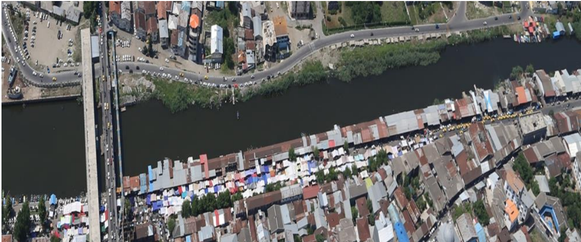
Figure 4.24, An aerial view of corridor of old Saturday Bazaar with their crooked tin roof across the river
