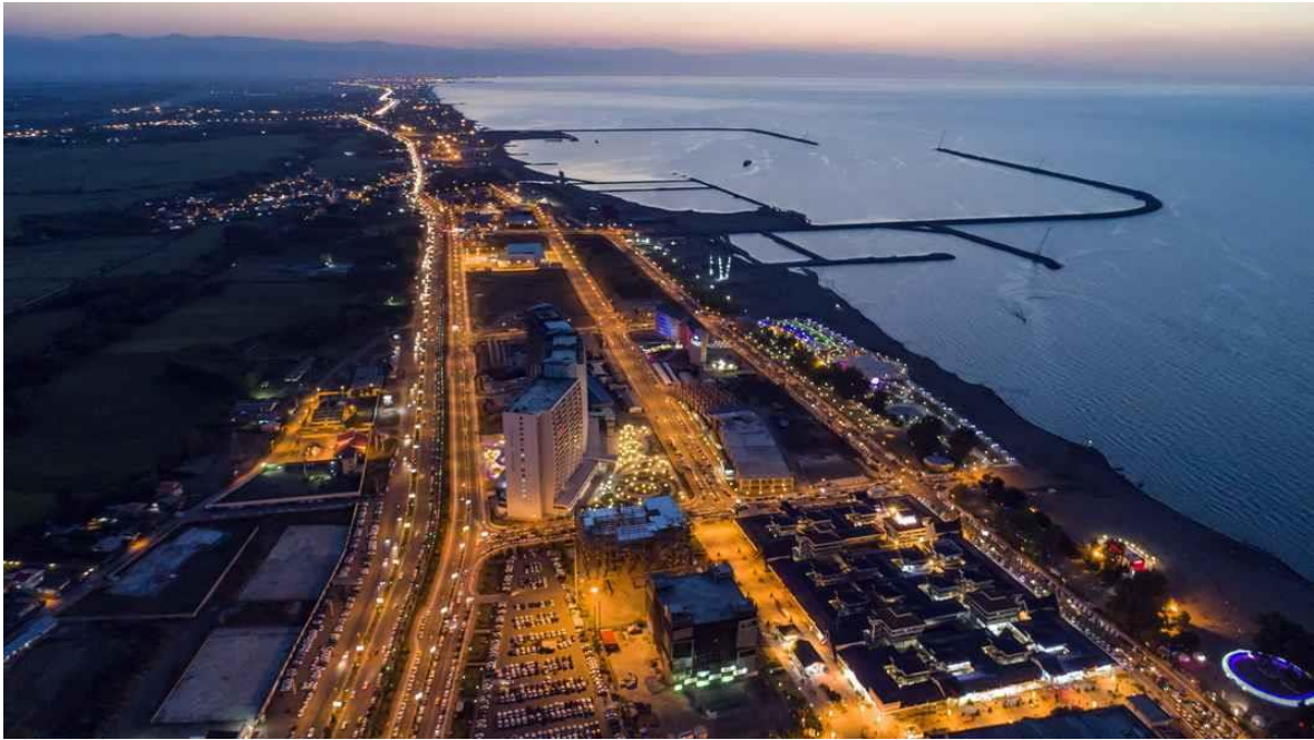
Figure 4.6 A view of Caspian Port Complex. Source ( http://caspianportcomplex.com )
