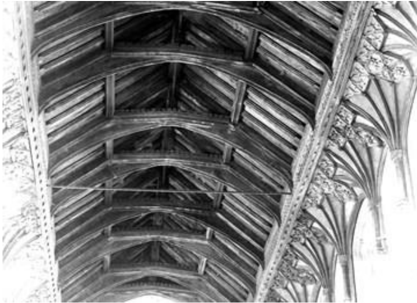
Figure 51 Ceiling at Church of St Michael the Archangel, Framlingham, Suffolk.
