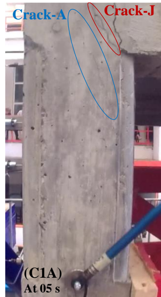
Figure 4.14: Shear crack (crack-A) developing in column C1A during 1.6g test for the CC-EQ building
