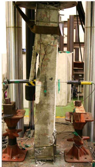
Figure 2.4: Failure mode of RC columns with tyre rubber particles (Son et al., 2011)
