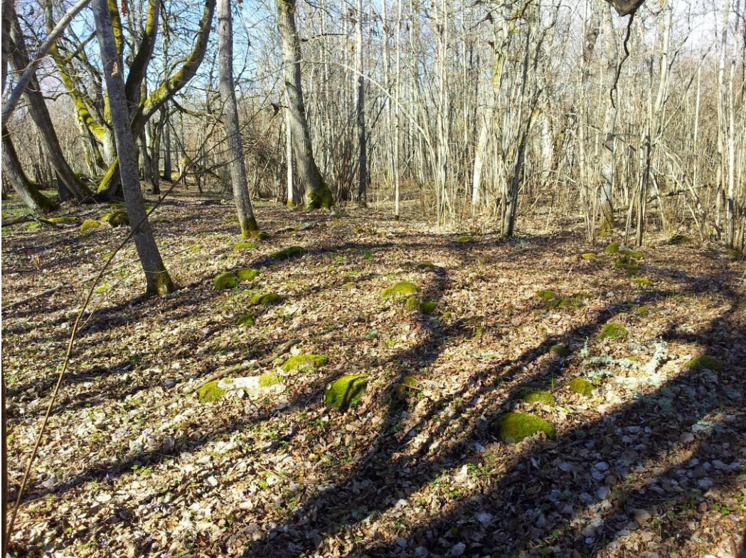
Figure 5.29. Section I-5, view from E (2014).
