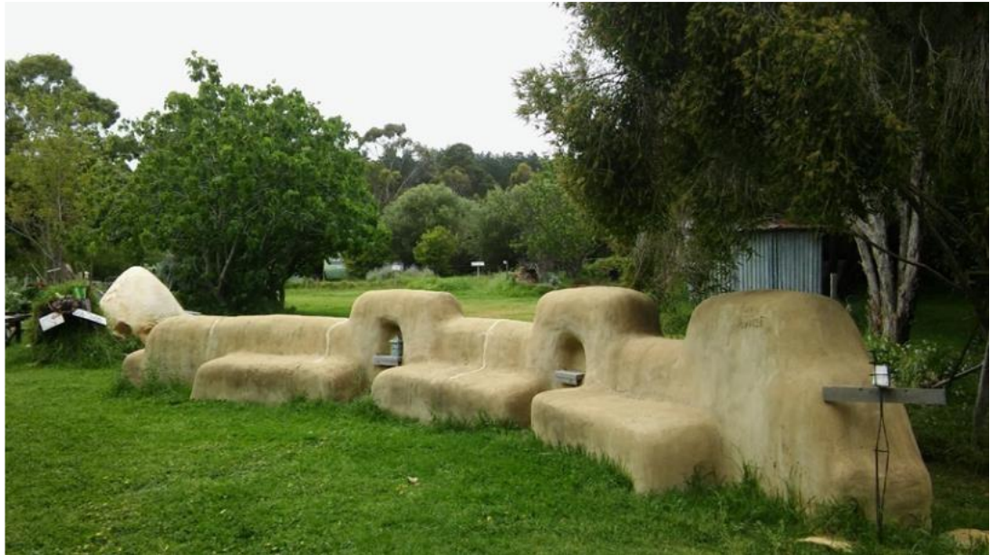
Figure 24: Cob seating area. Vernacular material, democratised building skill, communal area, natural setting, Fairharvest Farm. Photograph by author Oct 2017
