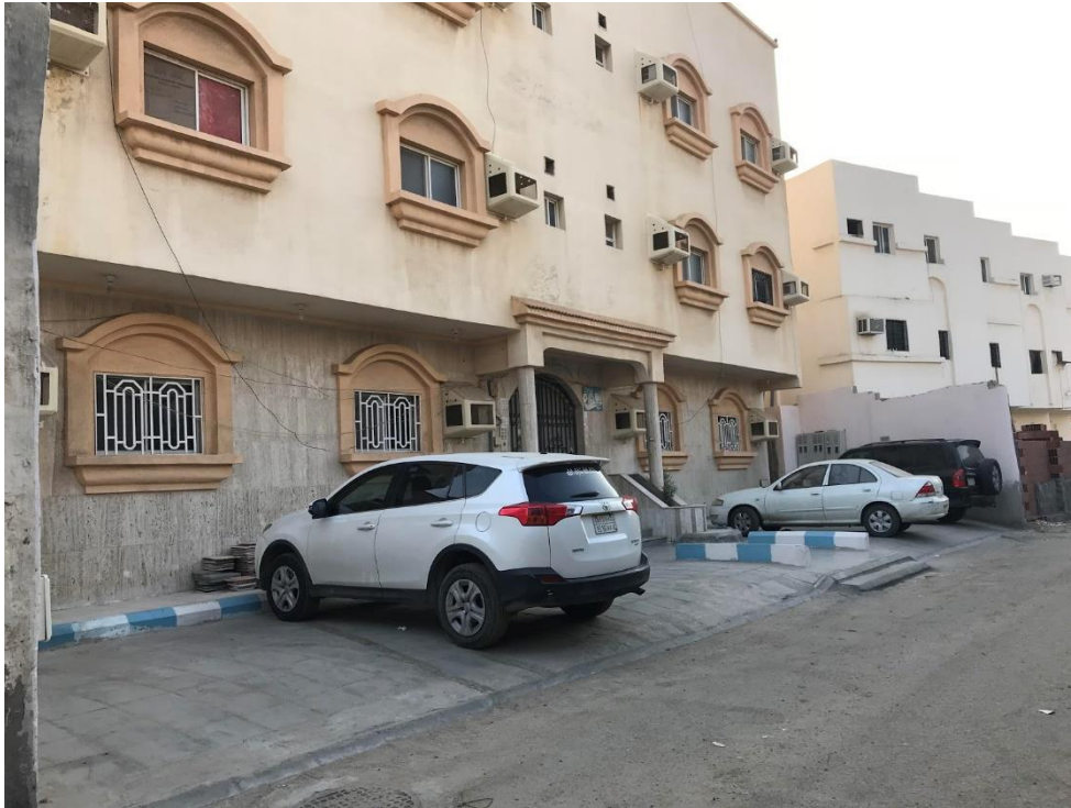
Picture 5.3: Houses of residents of Sifran hara (a tribal hara), built with concrete and steel and renovated with a modern design. The Street is wide and paved and has specified parking spaces.
