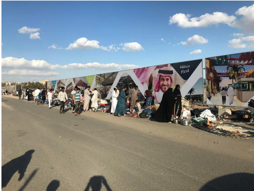
Picture 7.3: After the demolition, was complete, local people still continued their activities. Date: 2019
