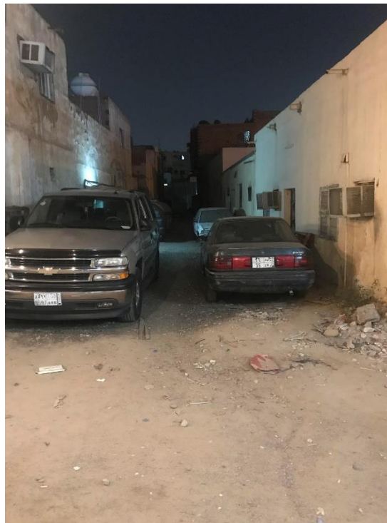
Picture 5.4: Typical houses in the Kilo 6 area looking neglected and no signs of modern design are visible. The street is narrow with no pavement and no parking spaces.
