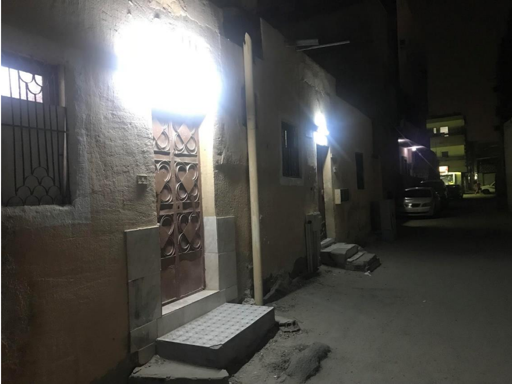
Picture 5.8: Attached houses located close to Jihnan hara. They look upgraded: good paintwork and well lighting, a semi-paved street with no leaks or cracks, and electricity cables are covered.
