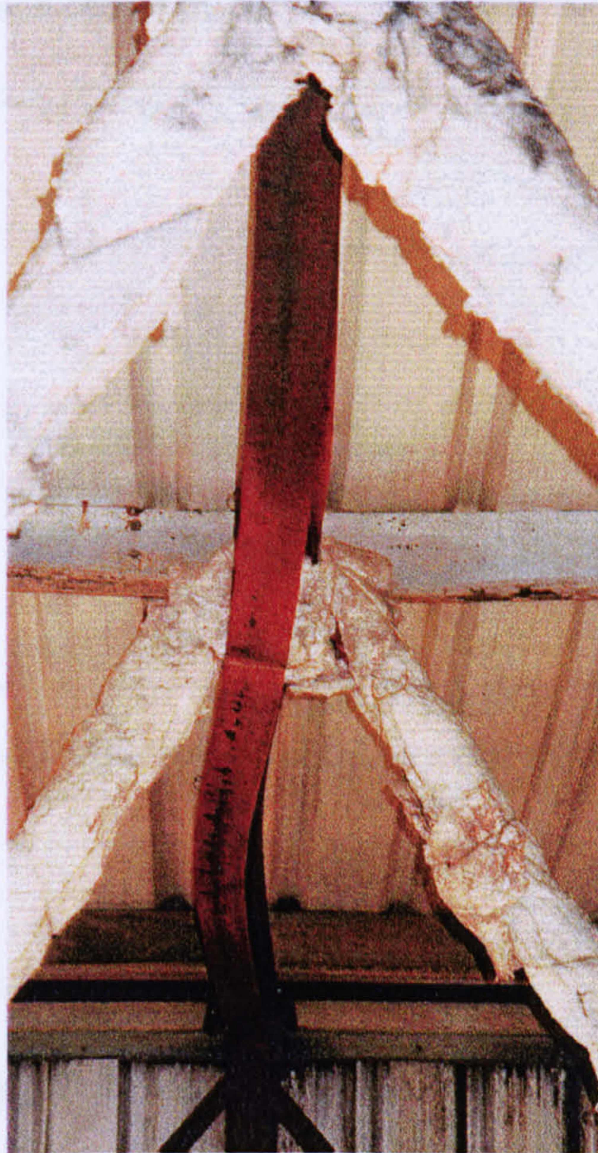
Figure 4.18 Lateral deformation of rafter from the second fire test
