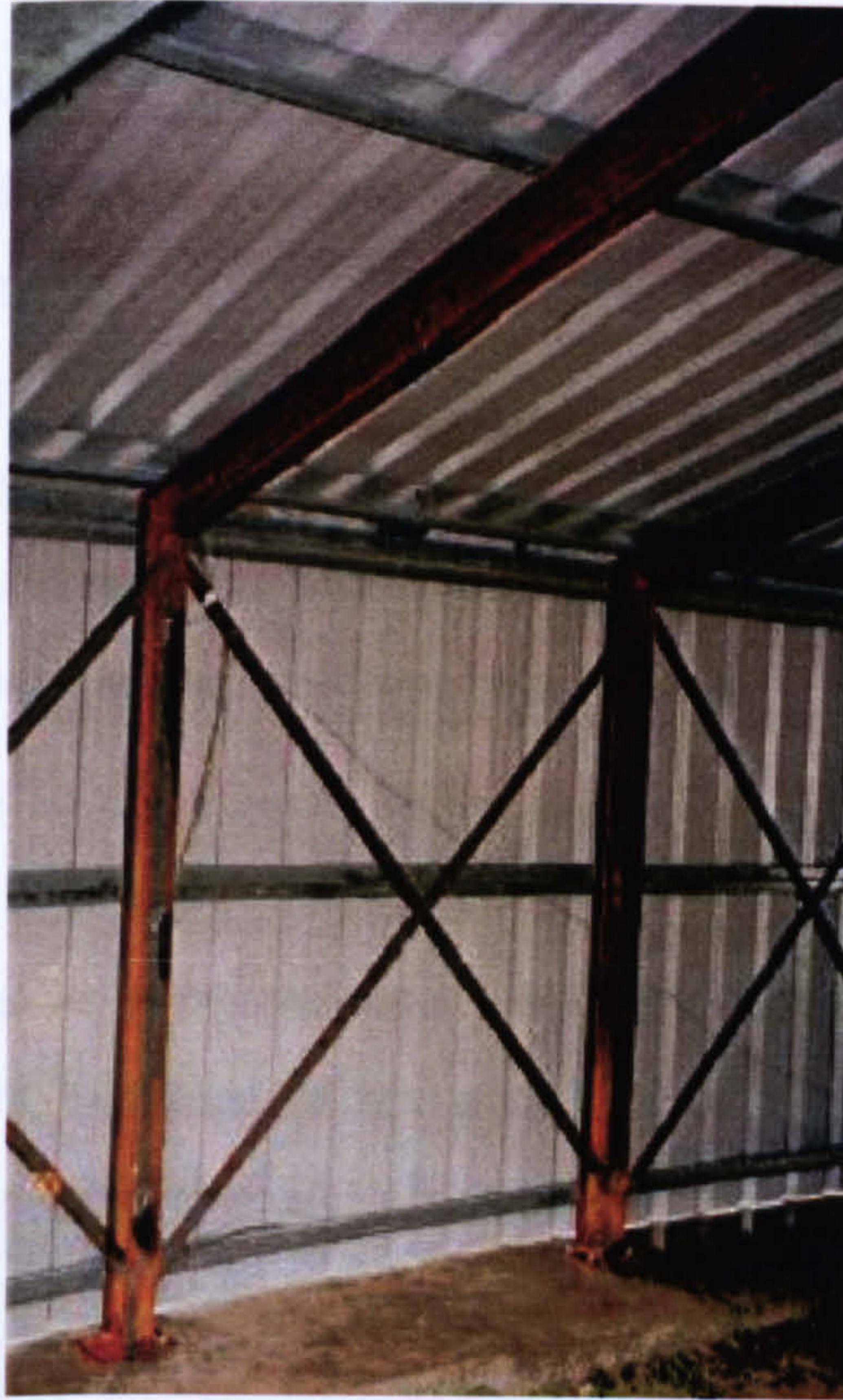
Figure 4.6 Lateral support system
