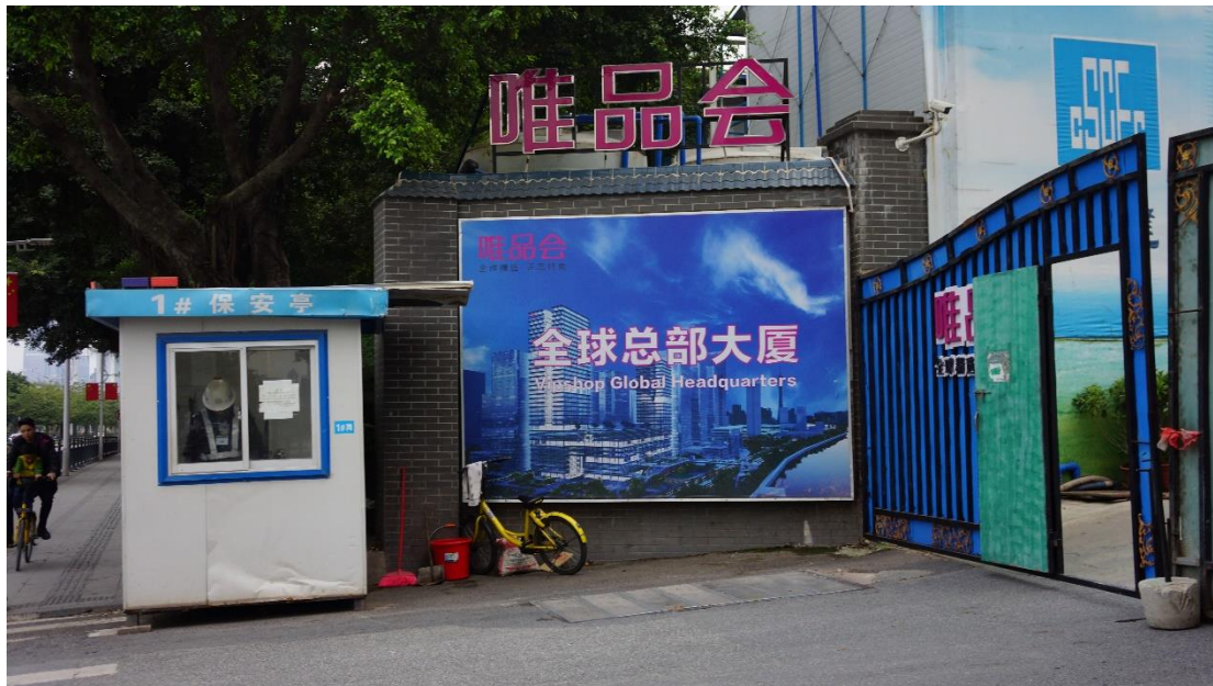
Figure 5-13 Construction site of the Vipshop company.
