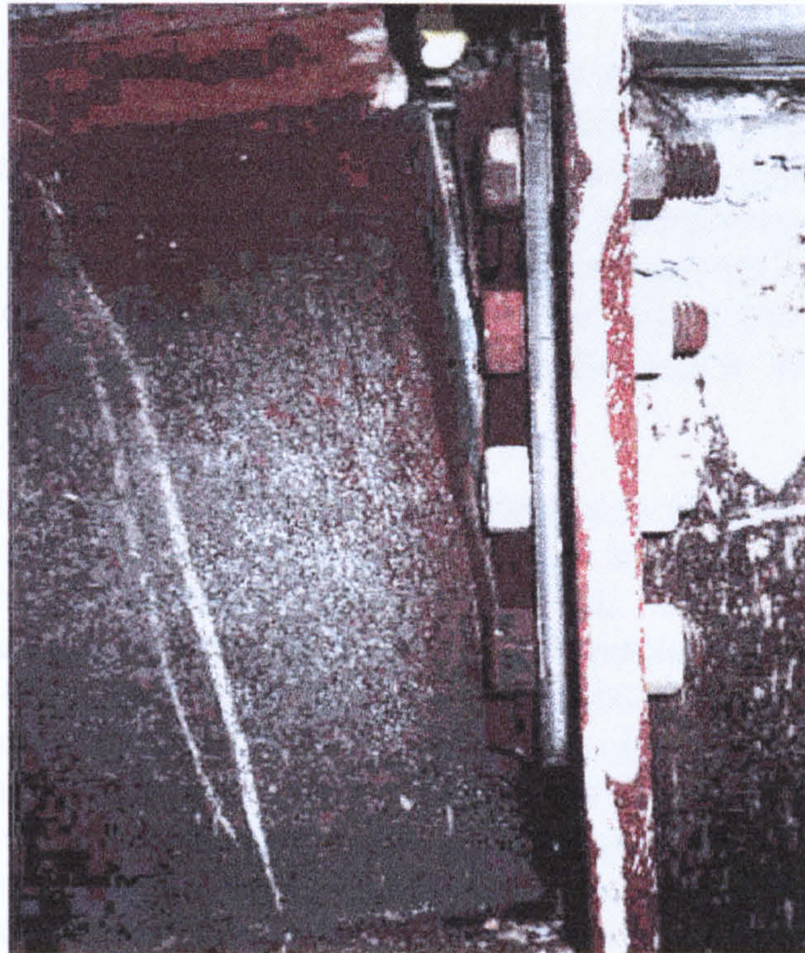
Figure 4.5: Elevated Temperature End-Plate Failure Mode for Group 4
