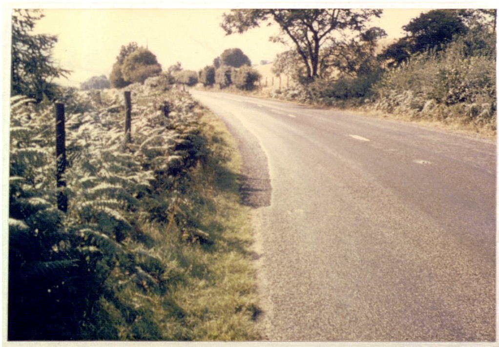
Plate No. 7.47 Repairs to the A57 road due to movements of the landslide at Rowlee Pasture.
