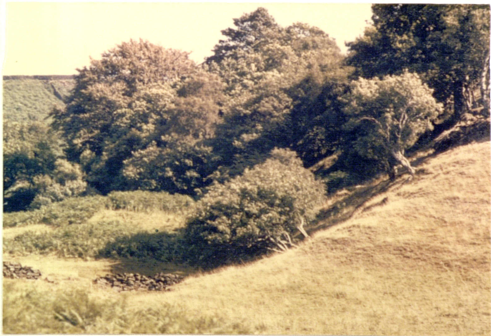
Plate No. 7.34 Minor scarp on the eastern side of Bretton Clough with evidence of recent instability
