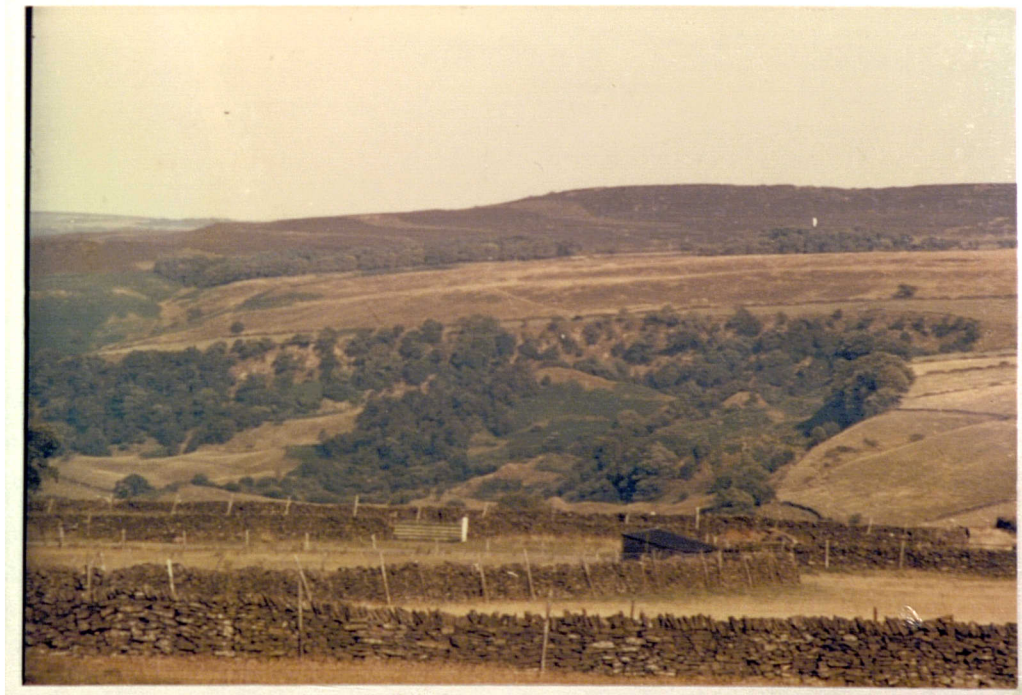
Plate No. 7.32 Eastern landslip at Bretton Clough - general view.
