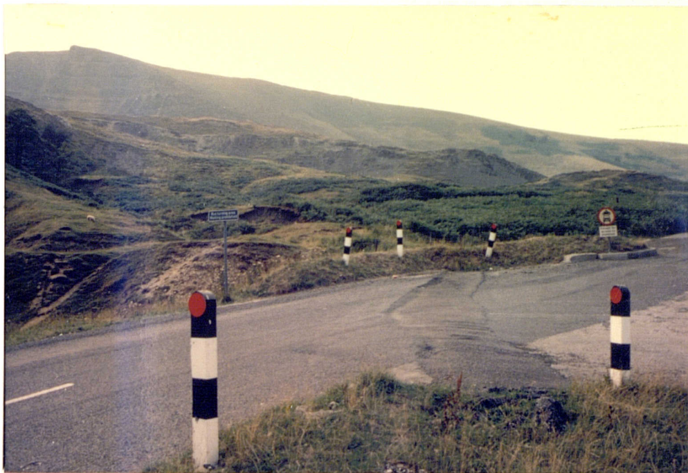
Plate No. 7.8 Hummocky ground at the foot of main unit. Recent downward movement of lower southern edge of the road in January 1983.
