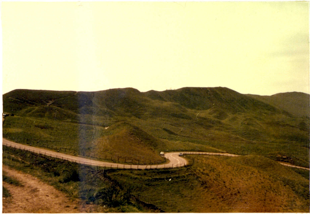
Plate No. 7.13 Main scarp and main unit landslip at Rushup Edge.
