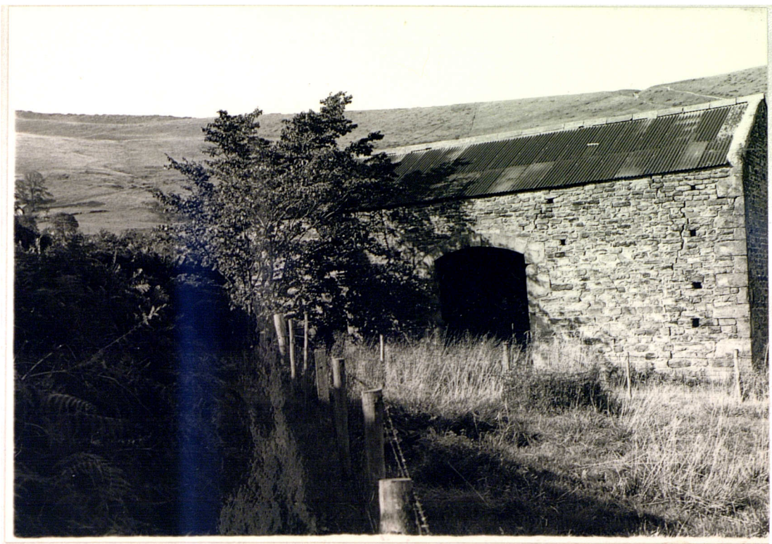
Plate No. 7.10 Blacketlay Barn before March 1983.
