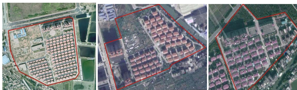
Figure 3.5 Redeveloped villages (Yufengxincun, Nanronghuayuan and Haiyuyuan)
