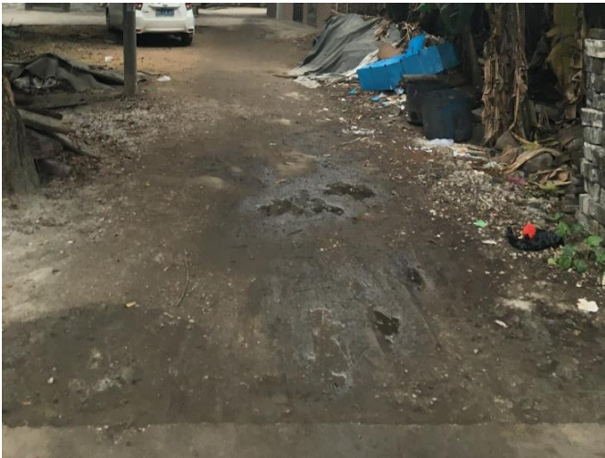
1 Heavily littered with substantial accumulations
