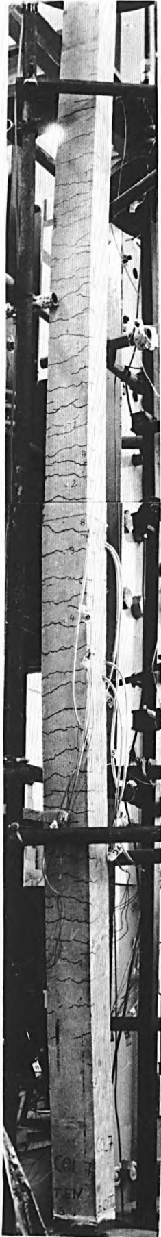
Fig.5.10 Typical crack pattern (C7).
