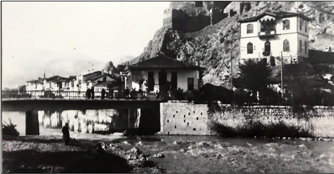
Fig. 5.42. Picture of a new Helkis (Hukümet) bridge during the construction of a new bridge in 1940 (Menc, 2018, p. 117).
