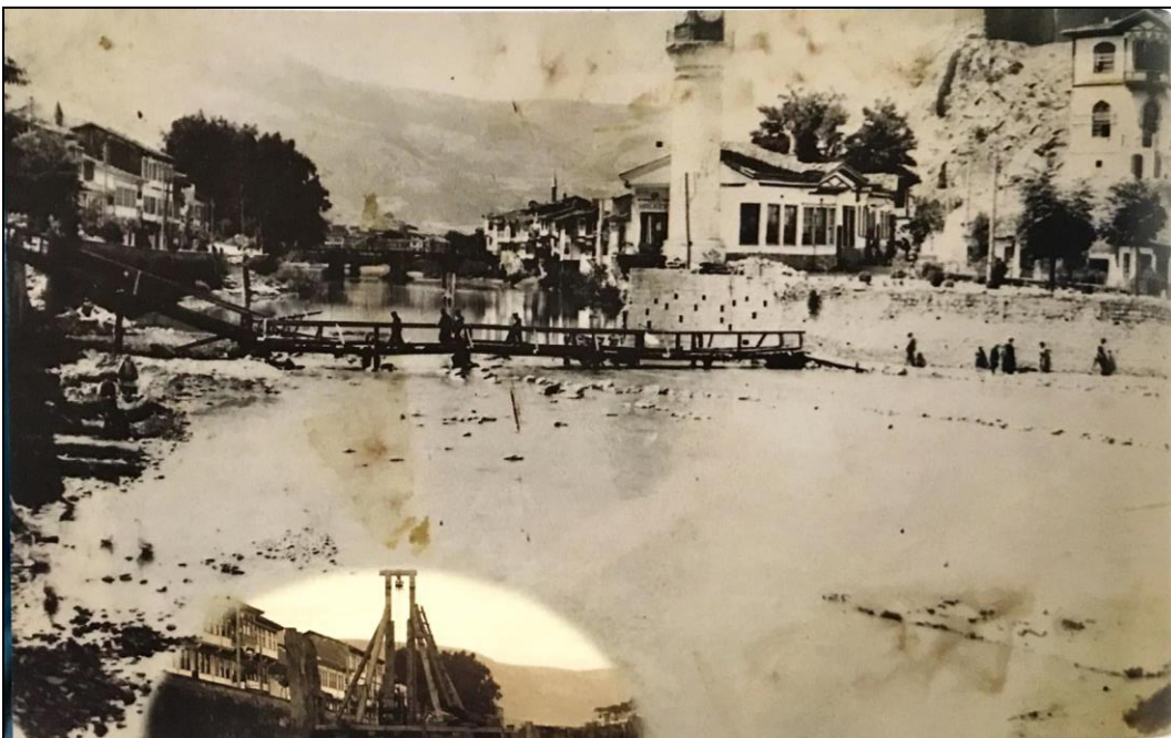
Fig. 5.41. Picture of a temporary bridge during the construction of a new bridge (Menc, 2018, p. 116).
