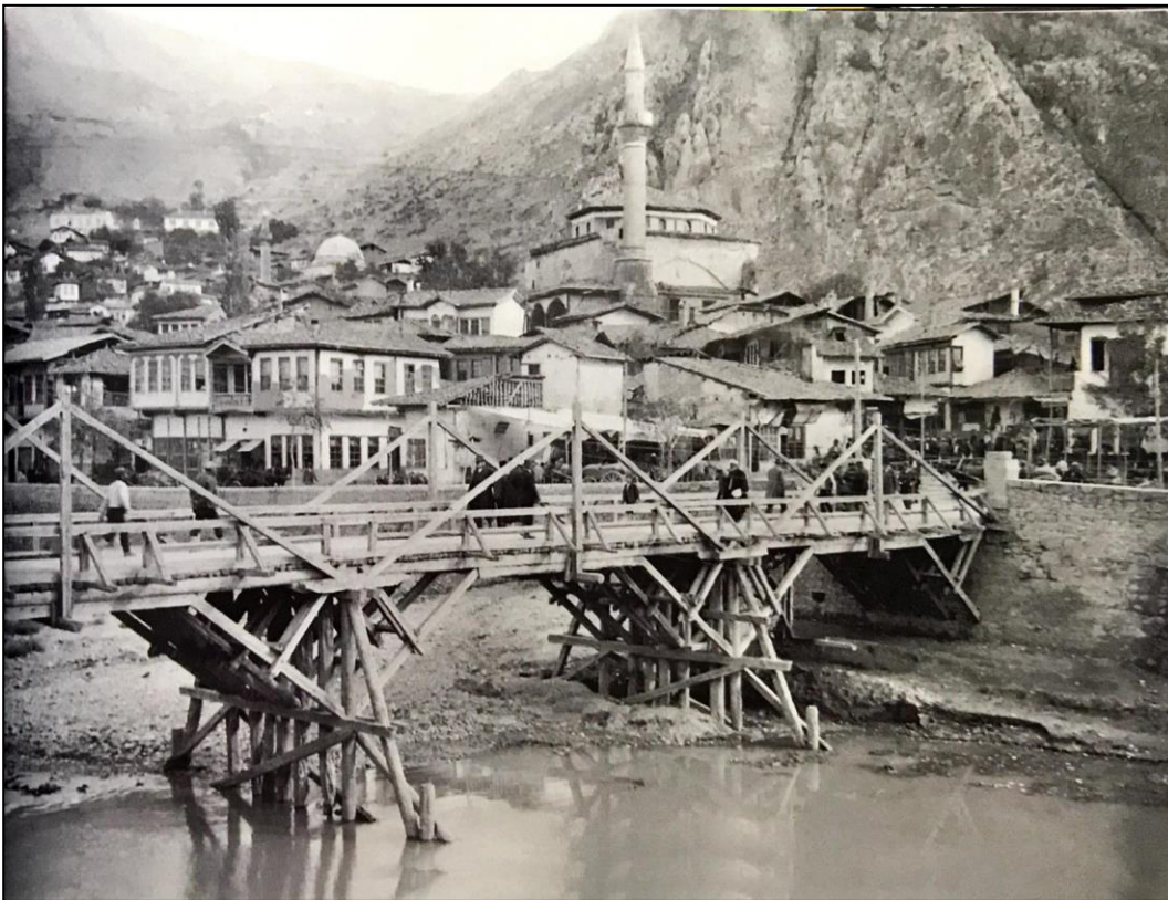
Fig. 5.40. Picture of Helkis Bridge in 1930 by Albert Gabriel (Menc, 2018, p. 113).
