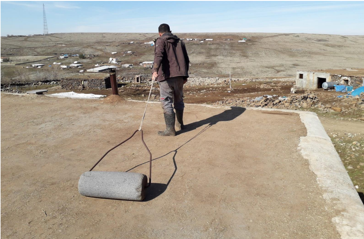
Fig. 5.47. A man using 'Log Tasi' for flat earth roof maintenance (Kurt, 2020).
