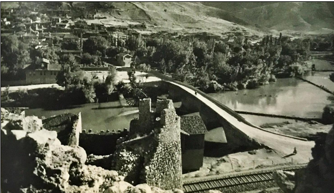
Fig. 5.43. Picture of a Meydan Bridge (Menc, 2018, p. 119).
