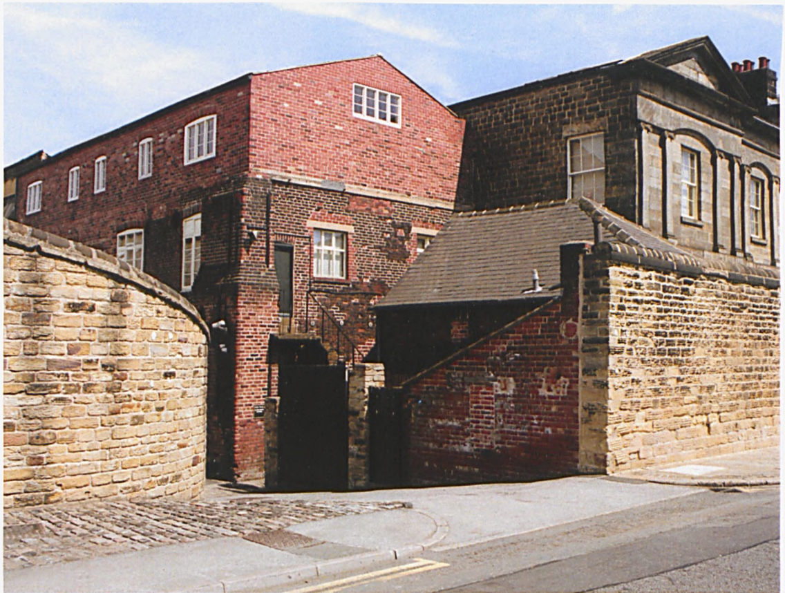
Fig. 3.76 Additional grinding wheels (left) were built at the side of the original courtyard in the early 1830s. Note the use of 'grindle cokes' as coping stones (author).
