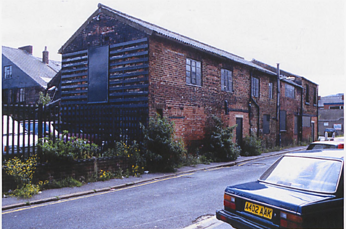
Fig. 2.55 Photograph of the buildings remaining on the site in 2002 (author).
