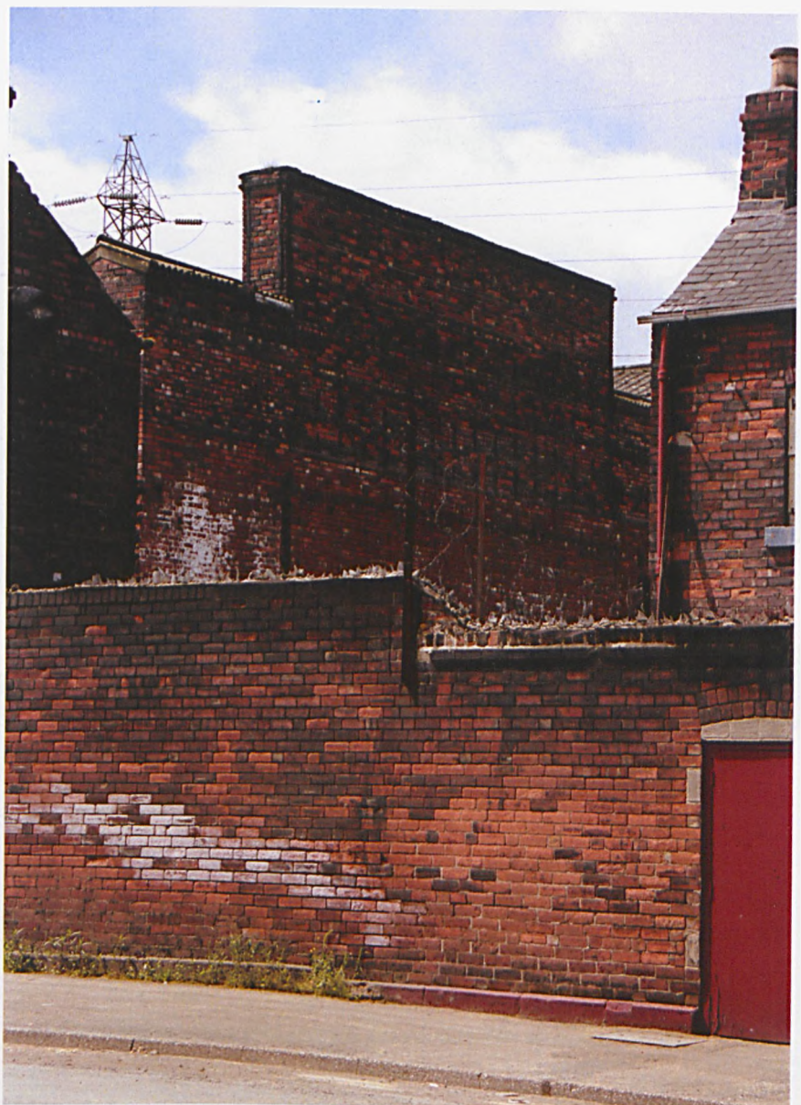
Figs 1.79 (top) and 1.80 Surviving steelworks buildings at Coleridge Road, including the porter's house, offices and warehouse and the melting shop behind (author).
