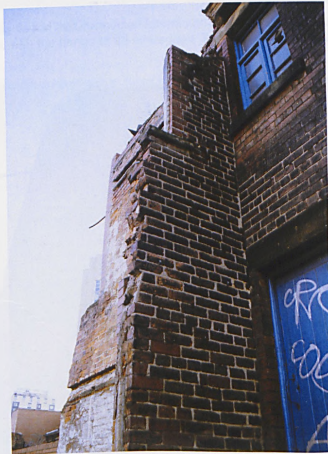
Fig. 4.95 Detail of partly demolished facade of Wells' Wheel, with partial survival of two window openings and lintels. The springing of the vaults is visible behind (author).
