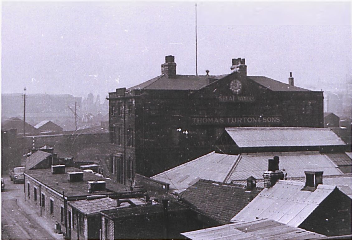
Fig. 3.60 Photograph of the warehouse at the Sheaf Works, looking towards Sheffield centre. Lightweight sheds had come to occupy most of the site (SCL).
