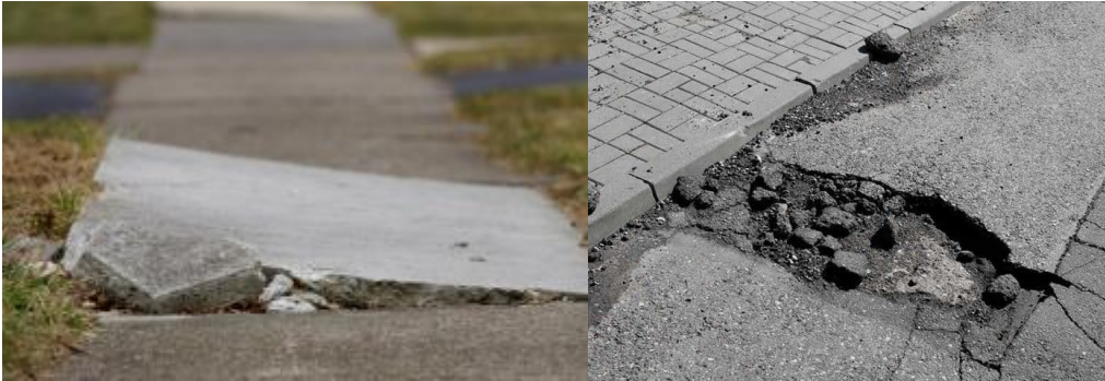
Figure 2.11. Uneven surface on the pavement may lead to a trip or fall. (Photographs by the author).
