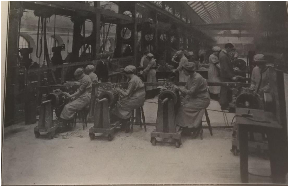
Figure 26 Armatures in course winding at Metropolitan-Vickers 1921 473
