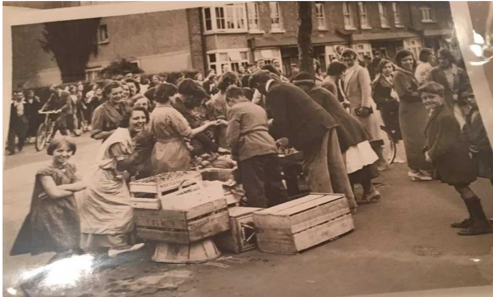
Figure 15 Women Striking at Mullard's Radio Valve Factory 394
