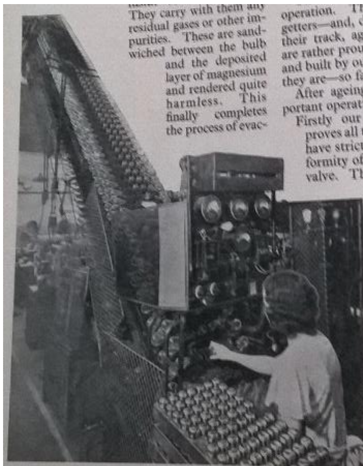
Figure 17 Automatic escalators at Cossor Valve Works 1937 444
