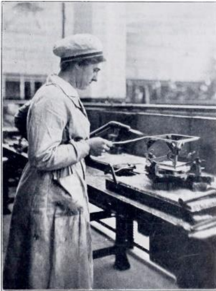
BRAZING THE FRAMEWORK OF COVER FOR A METER.
