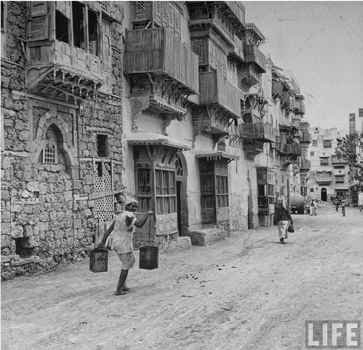
Figure 142: The houses in the old town of Jeddah were clustered in blocks in random arrangements due to the excessive heat and the need for air movement. Source: taken by the photographer Bob Landry for Life Magazine.
