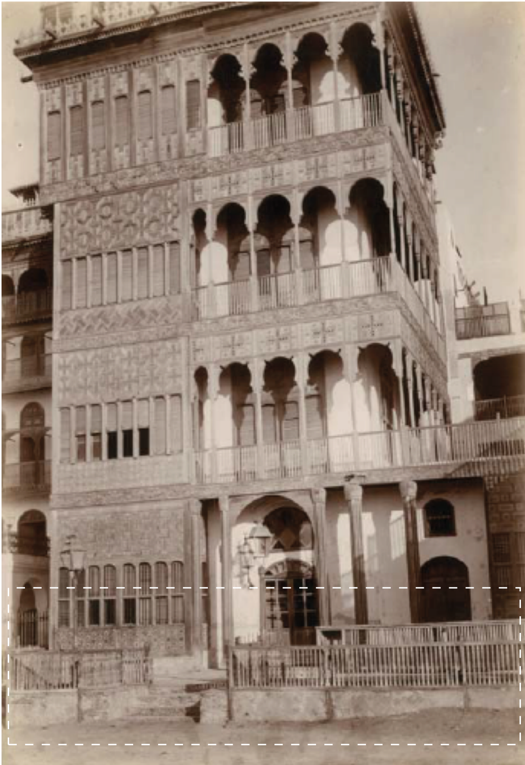
Figure 130: Photograph of the exterior of the Dutch Consulate, Jeddah c. 1910. Live edges in buildings affect the social interaction. Source: probably by Consul N. Scheltema. Cited in Vrolijk, Mols, 2016, p. 6.
