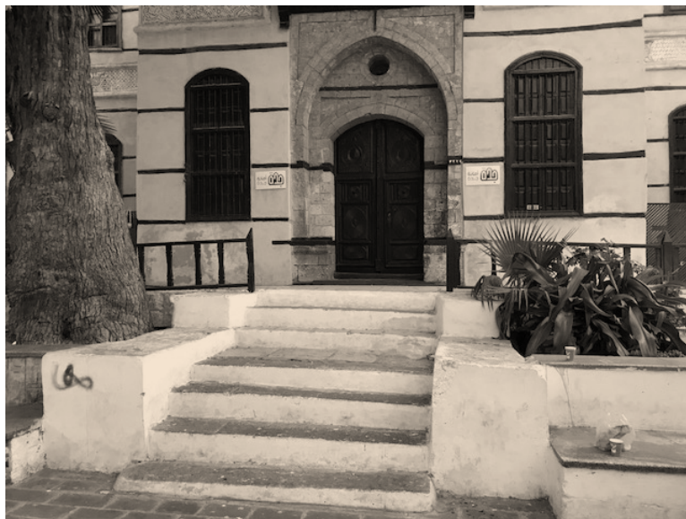
Figure 13: Stair seats. An example of stair seats in the old city of Jeddah.
