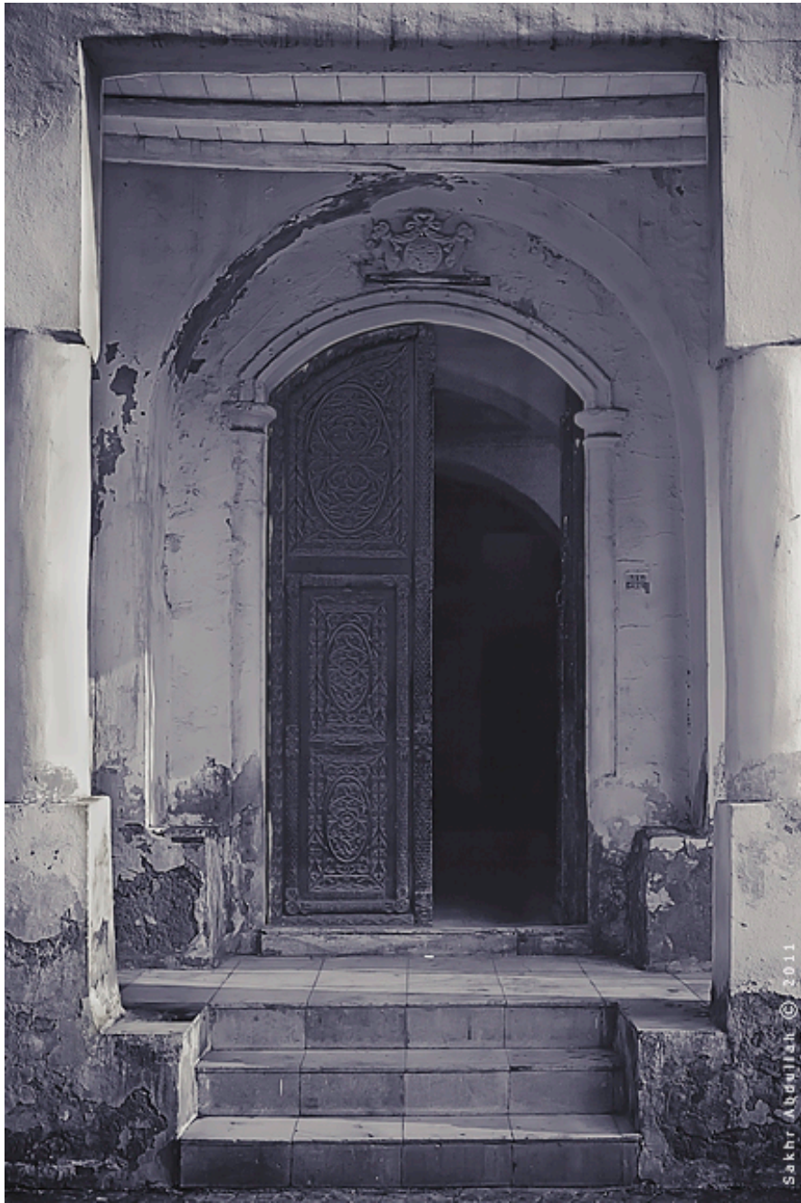
Figure 102: Al Ashgar House, main entrance, 2011. The door is more than 150 years old. Source: taken by Sakhr Abdullah, 2011. Al Ashgar House Door (Digital Image) (Viewed 26.09.2019).
