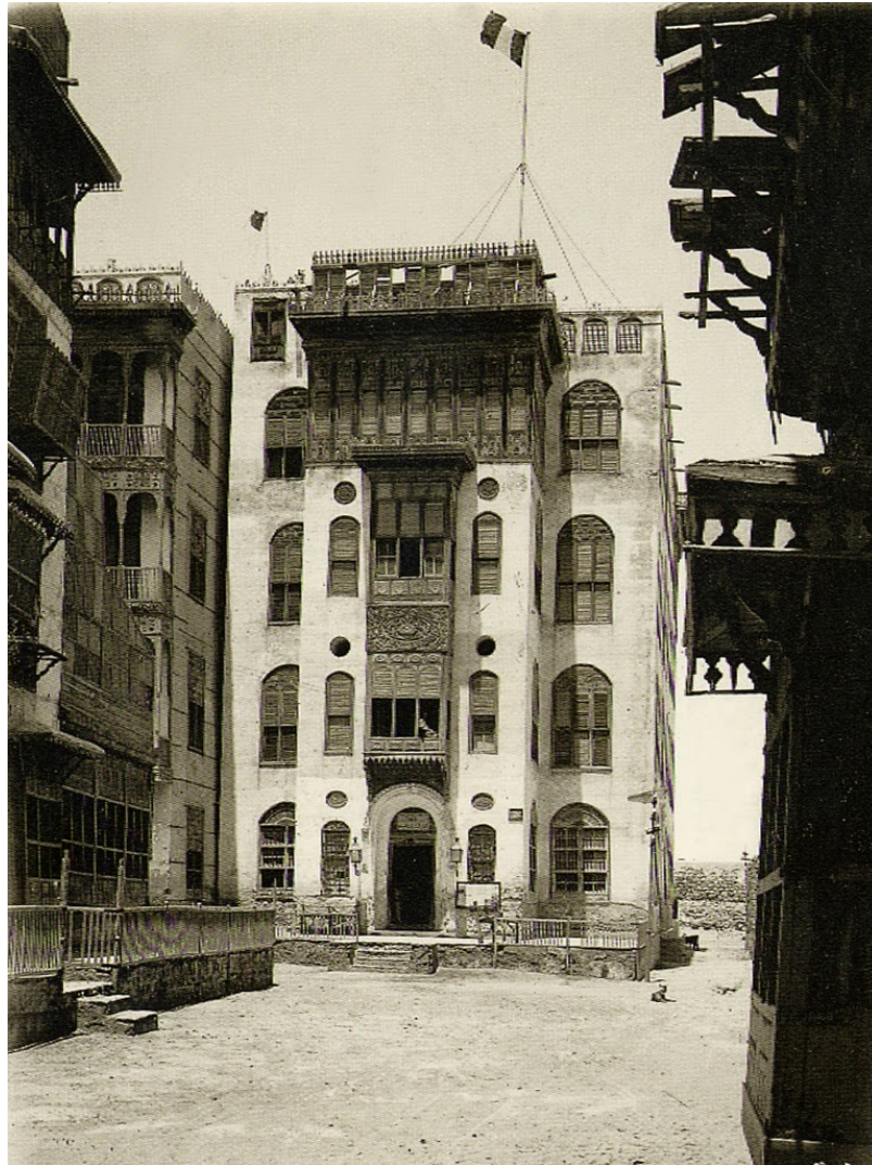
Figure 83: 1917 Barhat Faransa, located in Al Sham neighbourhood 1917. The building interacts primarily with the city via its façade. In this case the Dakkah works as an in-between space separating the private from the public. Source: http://lostopportunitiesandwastedtimes.blogspot.com/2014/05/blog-post.html (Viewed 12.09.2019).
