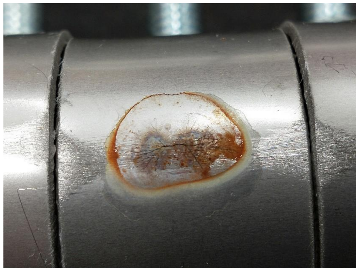
Figure 6.37 Discolouration indicating corrosion has initiated. The branching cracks characteristic of ASCC can be seen.
