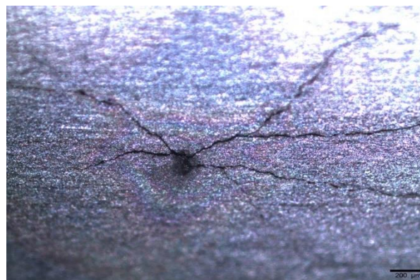
Figure 6.43 ASCC cracks on a rolled surface.
