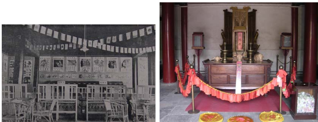
Figure 3.16 Interior of the Hall of God of Earth. (left) 1925, used as public library; (right) 2006, restored tablet of God of Earth. In front of it, there are cushions and a money box for donations from visitors praying. (Sources: (left) Ji Liu (刘骥), Jingzhao gongyuan jishi (京兆公园纪实 Authentic records of the Capital City Park) (Beijing: [unknown publisher], 1925)); (right) photo by author, July 2006)
