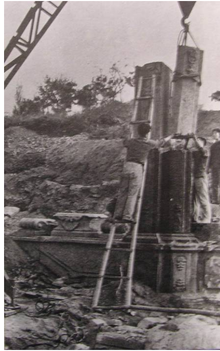
Figure 2.6 Anastylosis of monuments—reassembling architectural fragments found in Beijing University at their original place in Yuanmingyuan (1977) (Source: ‘Yuanmingyuan’, China Pictorial , 1981, No. 5)
