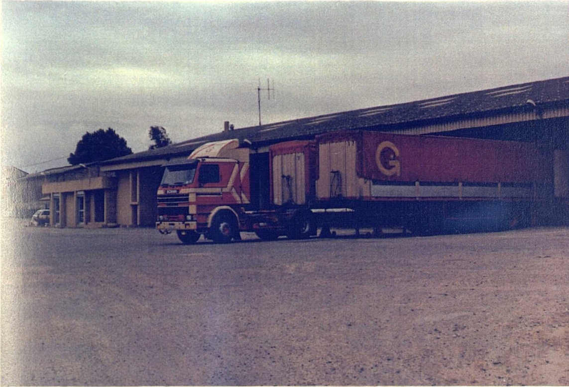
Figure 6.63 Transports Griset showing the 1978 extension and offices
