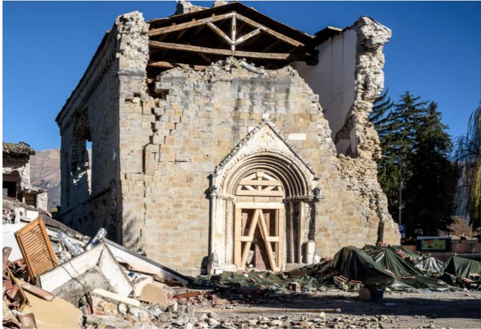
*Figure 7.1: Progression of the damage to the façade of Sant'Agostino after the earthquakes of August 24 and October 30, 2016. To note the lack of propping systems that caused further damage to the building (November 2016). @Antonio Ranesi*
