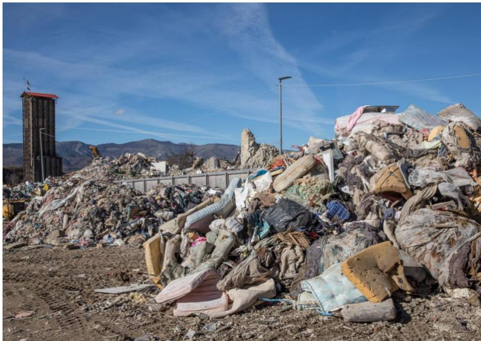
*Figure 7.2: A pile of rubber and mattress debris (November 2018). Before being removed, the rubble is divided by material. @Enrico Fontolan*
