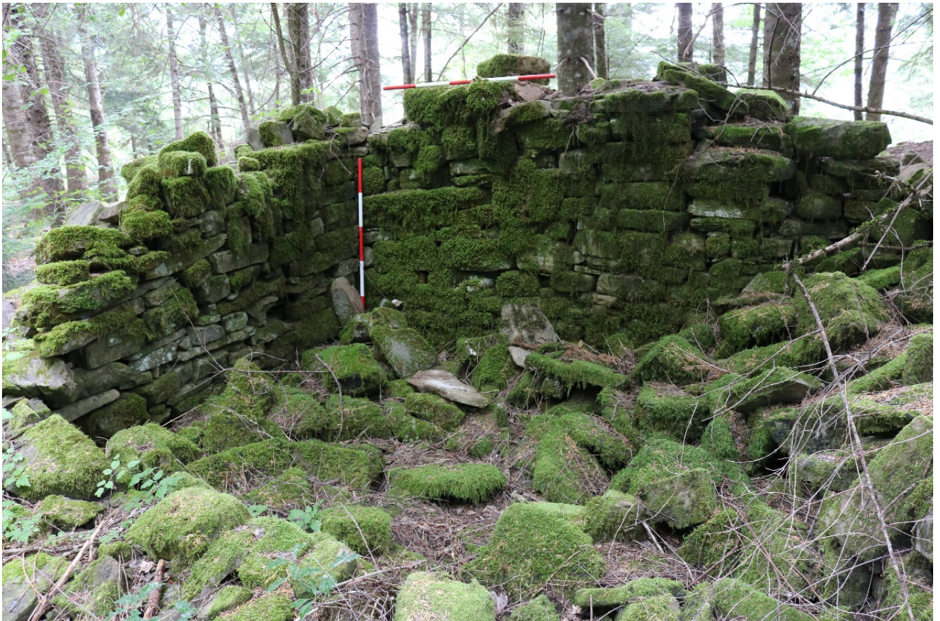
Figure 79: House in upper Koziakos village.
