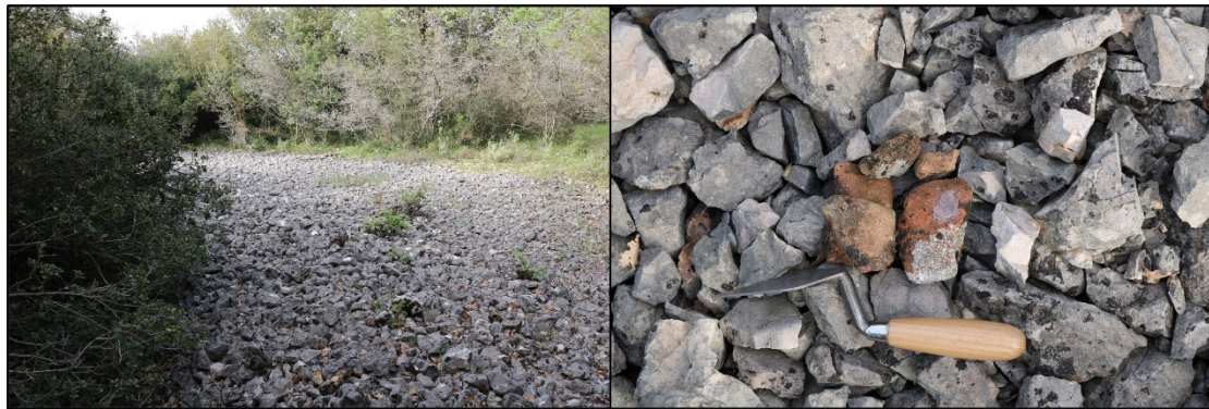
Figure 72: A collapsed structure in the area of the abandoned village.
