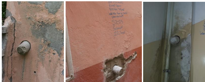
Figure 3-11: Concrete core samples taken from the building.
