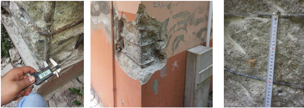
Figure 3-10: Cover removal and checking the columns' detailing.
