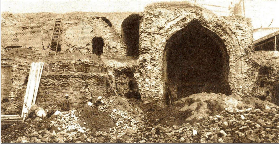
Figure 4.08: View of the iwan during removing the new layer of architecture. 64
