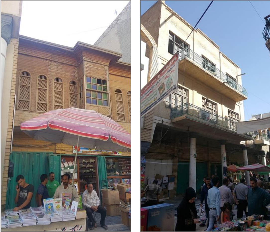
Figure 6.25: The listed heritage buildings in Al Mutanabi Street. 71
