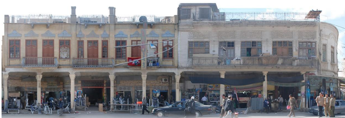
Figure 7.74: Two buildings prior to the rehabilitation in Al Rashid Street. 236
