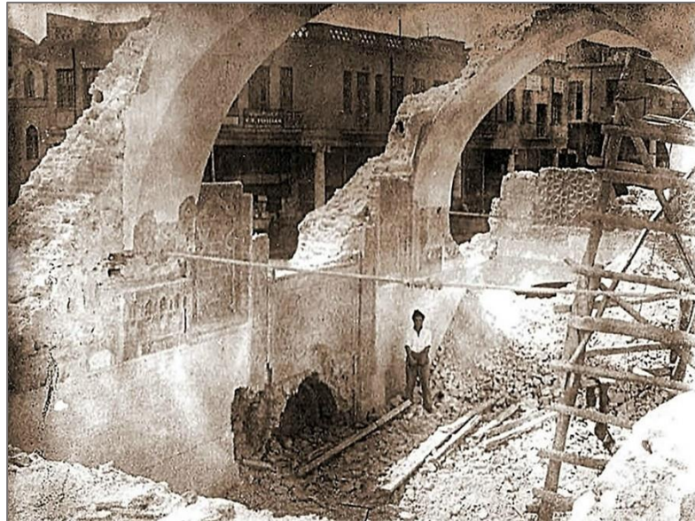
Figure 7.32: The demolition of Al-Madrasa al-Mirjaniya's musalla was stopped, but it was transformed to a ruin. 116
