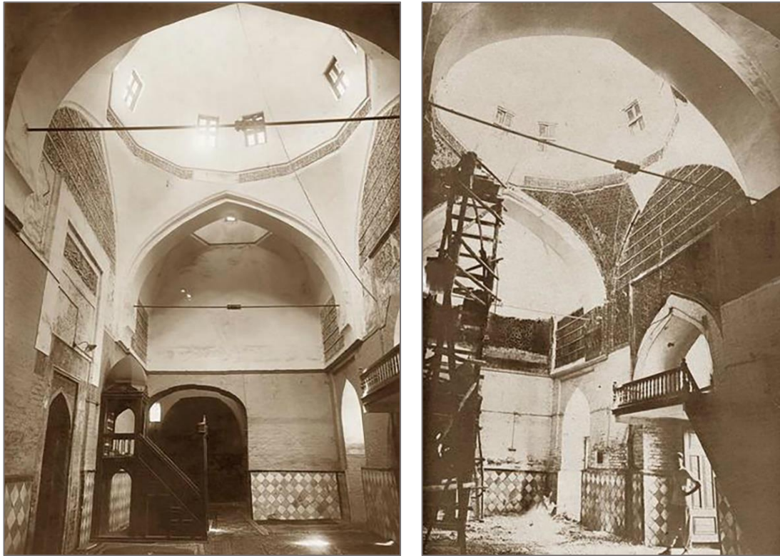
Left: Figure 7.29: Al-Madrasa al-Mirjaniya's musalla prior to commencing the demolition. 106 Right: figure 7.30: Splendid inscriptions and decorations were discovered under layers of plaster in the Al-Madrasa al-Mirjaniya's musalla after the start of demolition. 107
