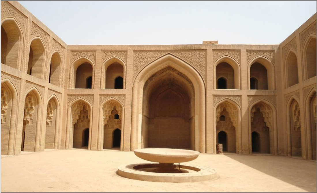
Figure 4.18: View of the eastern wing after the reconstruction of the first floor. 111
