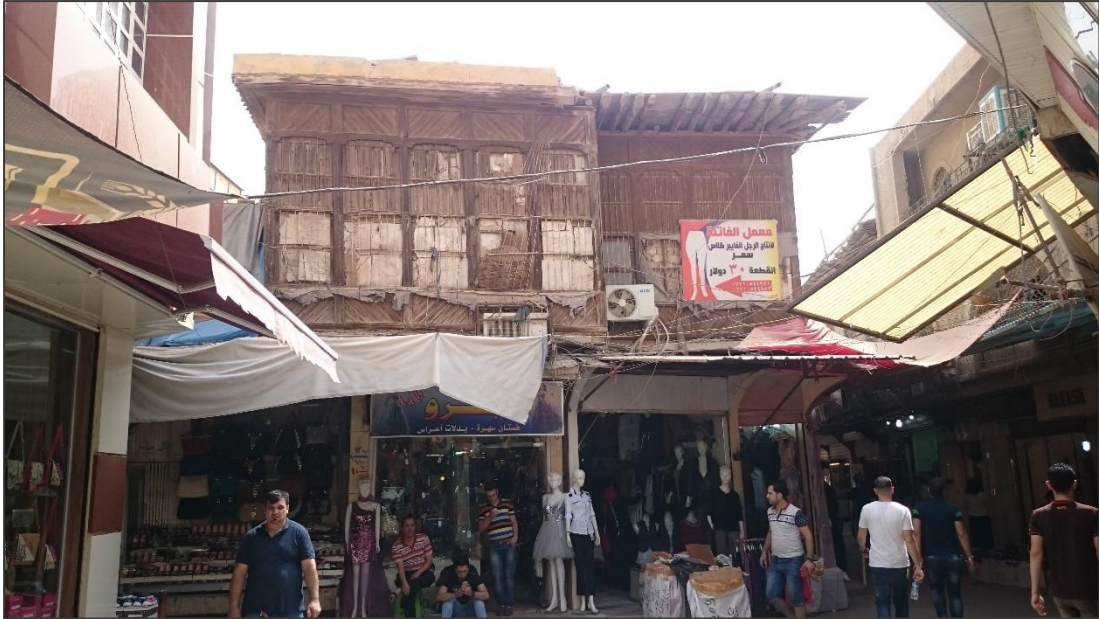
Figure 5.23: A Baghdadi traditional houses accommodates commercial use.
