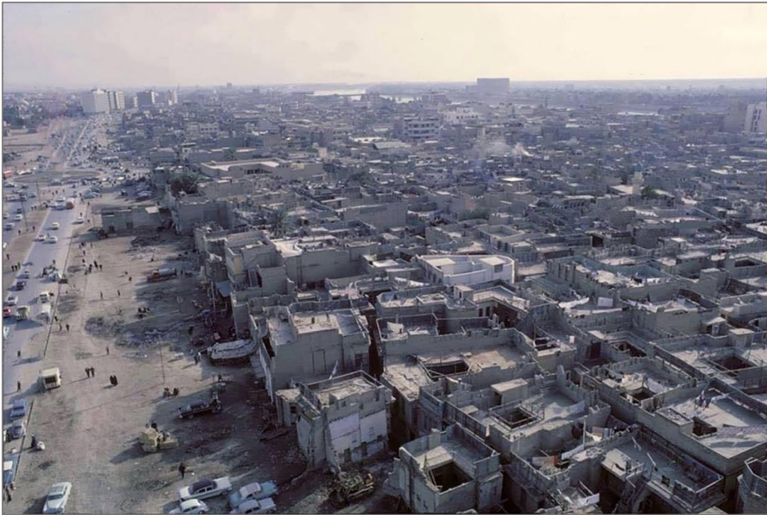
Figure 5.02: Khulafa Street after cutting back the historic fabric. 40
