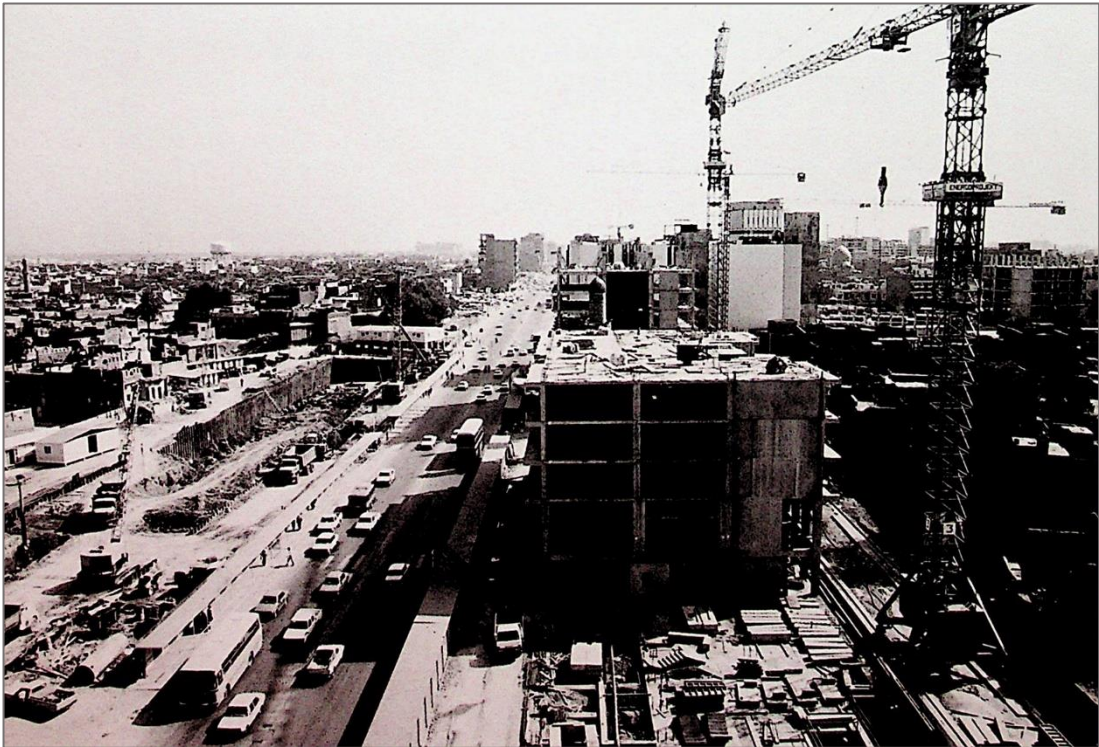
Figure 5.03: Constructing high rise buildings in Khulafa Street. 42
