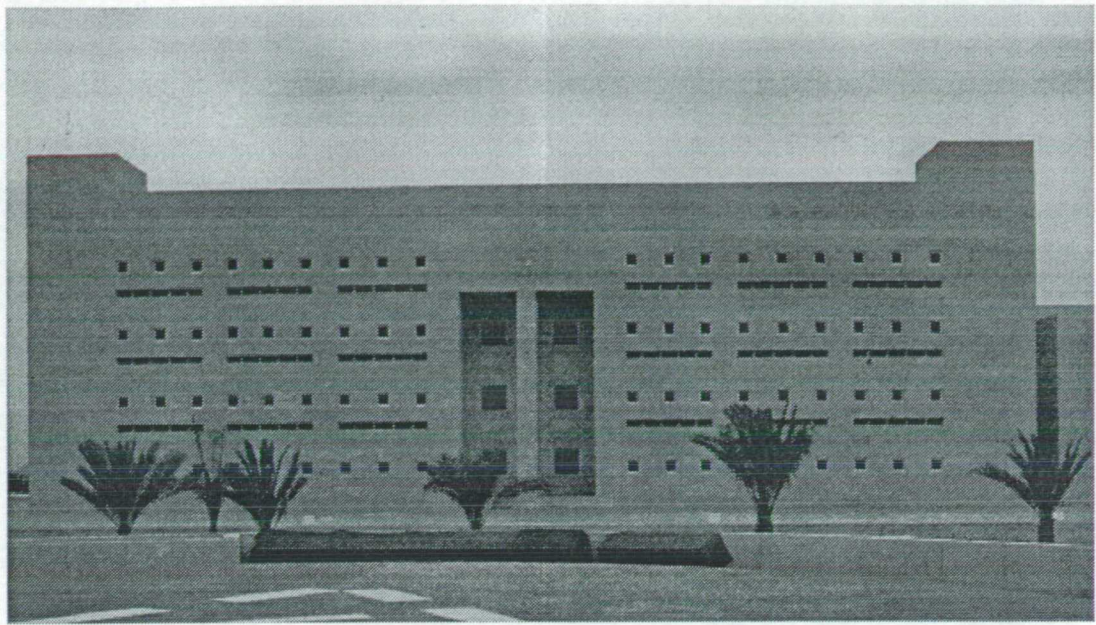
Figure 1.2 Another form of protection from direct sun radiation and heat gain is the use of small windows.
