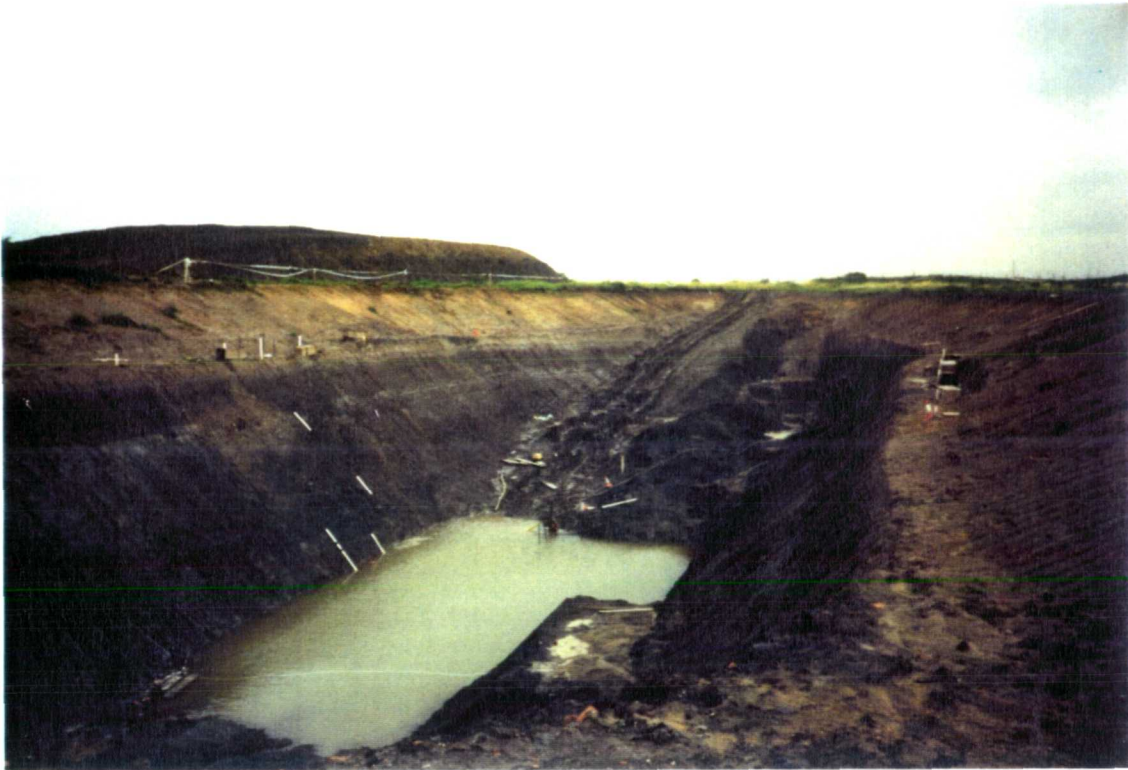
Figure 3.22 - View from south-west prior to backfilling excavation (31 July 1987)
