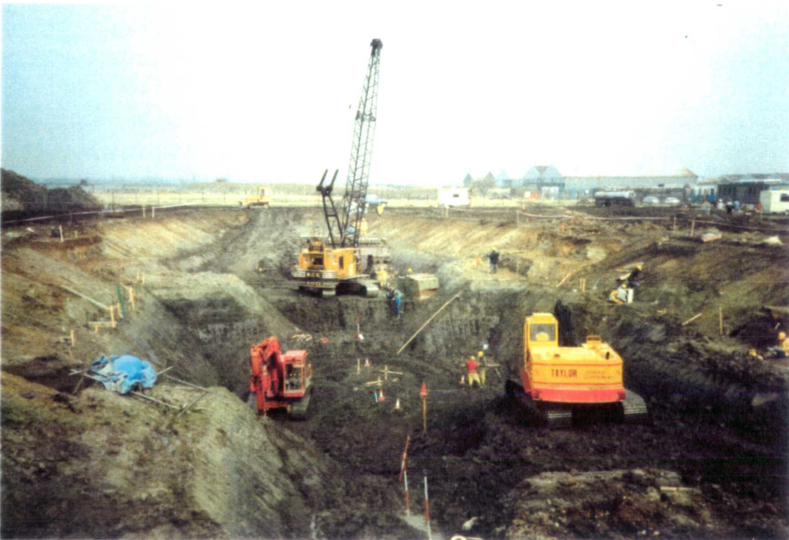
Figure 3.18 - View from south-west showing excavation at 5m depth (2 April 1987)
