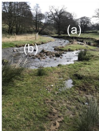
1. (a) Bank erosion and (b) gravel deposition
