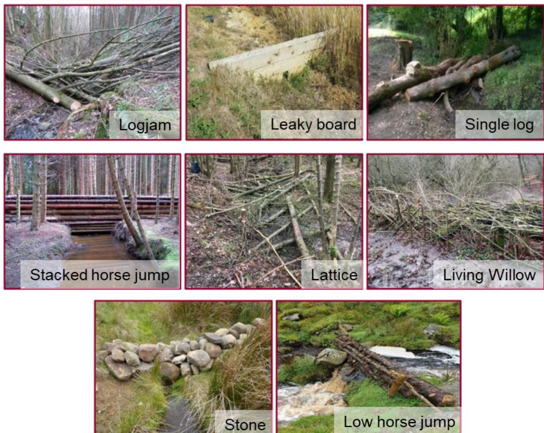
Figure 5.1: Variability in leaky barrier types. Modified diagram (names added) from JBA Trust (2020), p.2.
