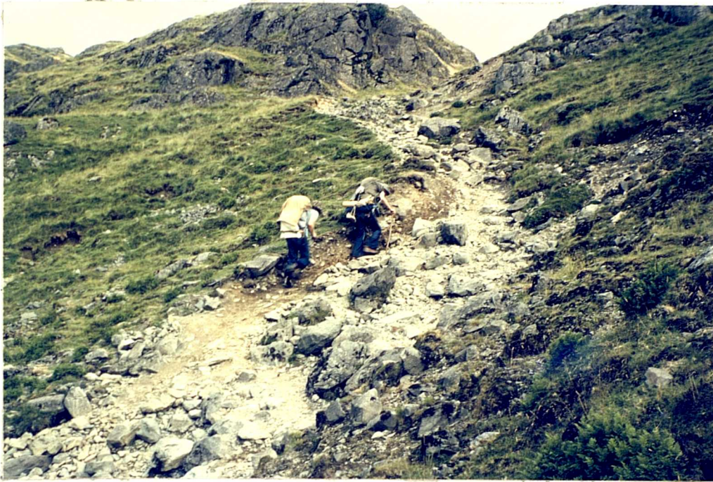
PLATE 5(a) Path erosion on Helvellyn (Wythburn, site 5)
