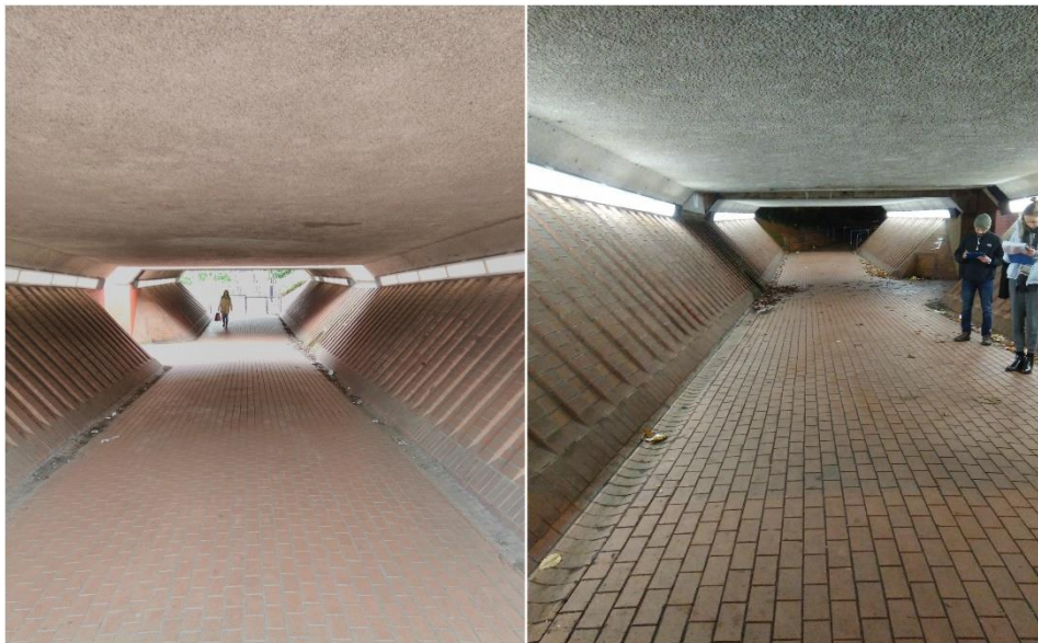
Figure 4. Pedestrian underpass during daytime and after-dark (R10).
