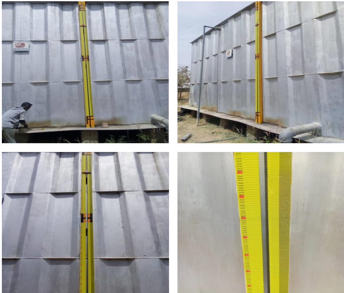
Plate 5.2: Tank gauge after installation
