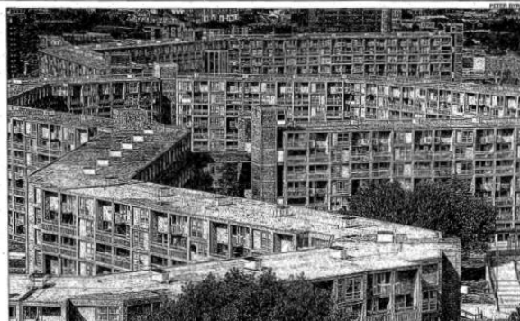
Park Hill in Sheffield, given Grade II* listed status by English Heritage, which calls it "a magnificent structure"
