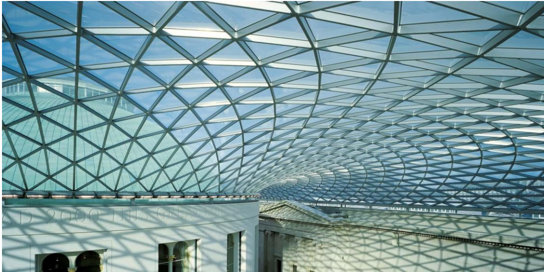
Figure 2.23 British museum roof made of triangular glass panels realized by Foster + Partners (available from fosterandpartners.com )
