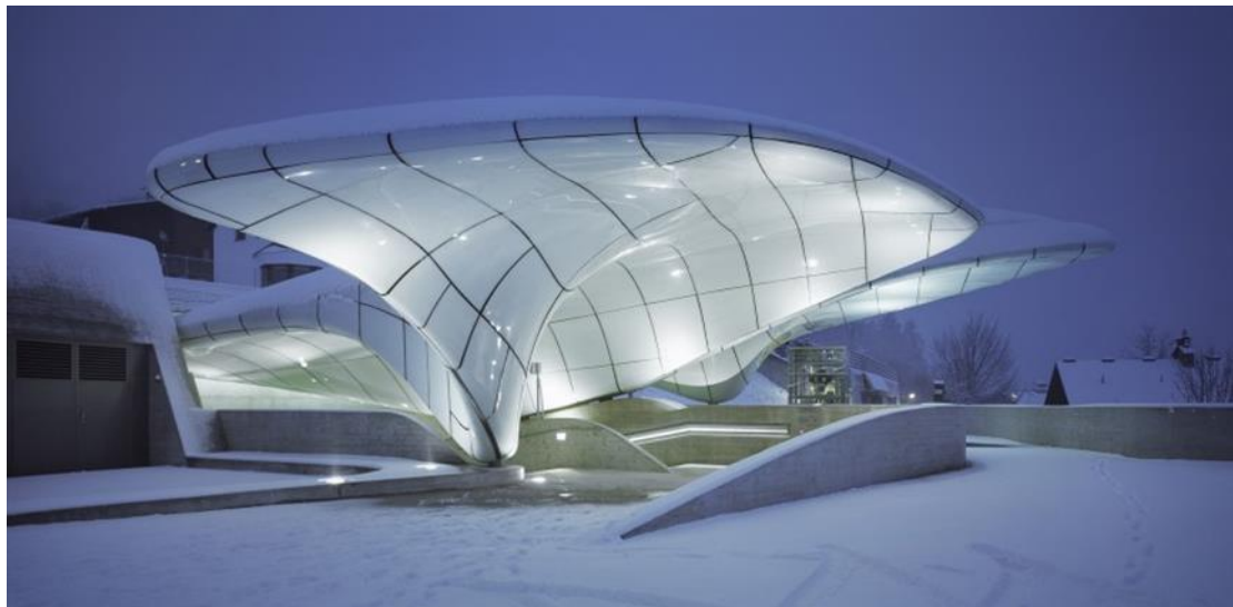
Figure 2.22 One of the four Zaha Hadid projects for the “Innsbrucker Nordkettenbahn” (Verner Huthmacher, available from bollinger-grohmann.com )
