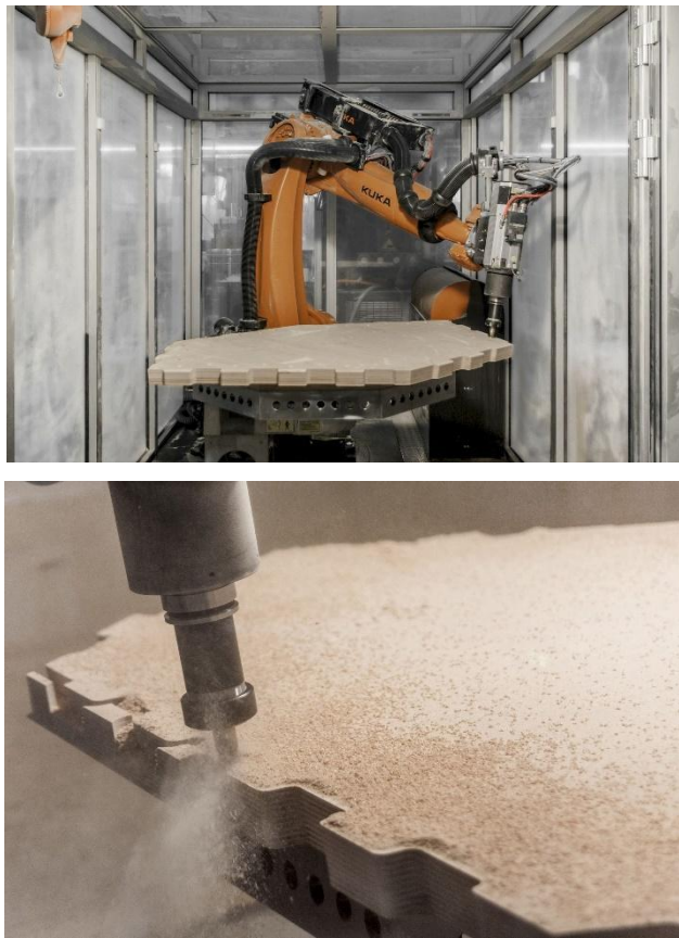
Figure 2.45 Finger joints realization through robotic arms for the Landesgartenschau Exhibition Hall (available from archdaily.com)
