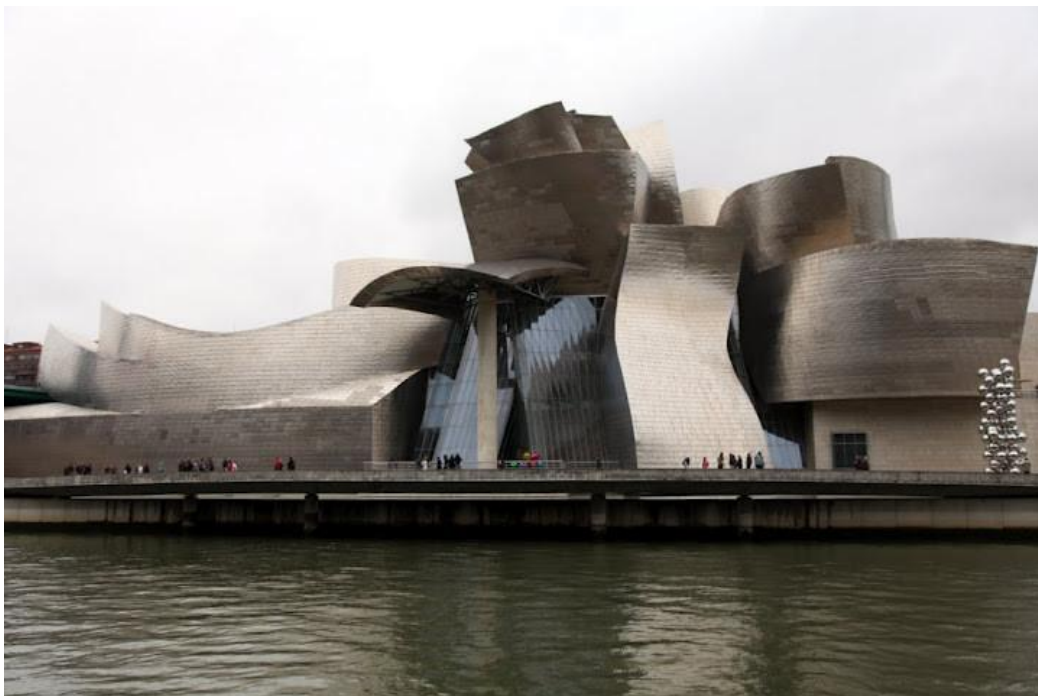
Figure 2.7 View of the Guggenheim Museum in Bilbao (available from archdaily.com)
