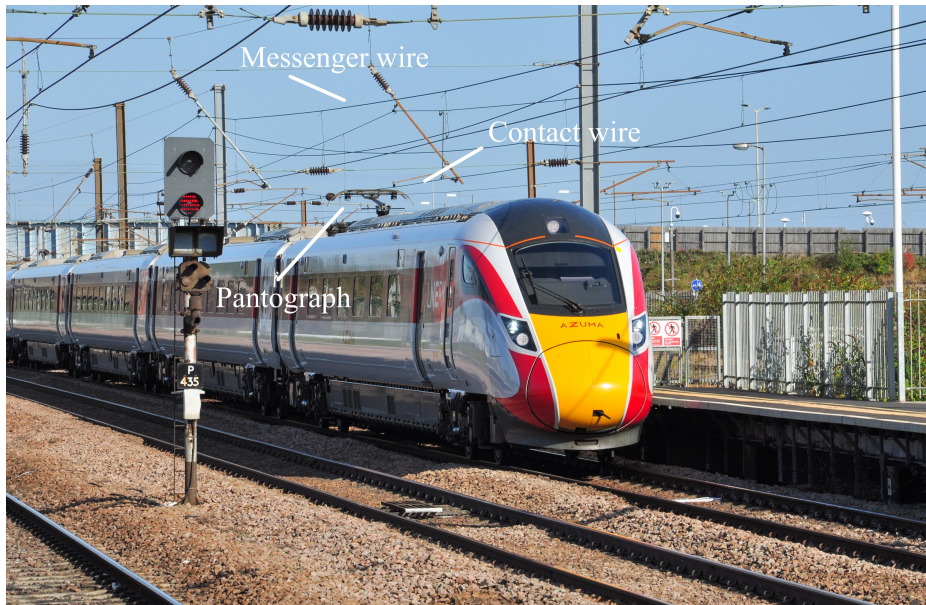
Fig. 1.1 Typical UK catenary pantograph interaction between the roof-mounted pantograph and overhead line equipment, Peterborough, UK. Image from [4].
