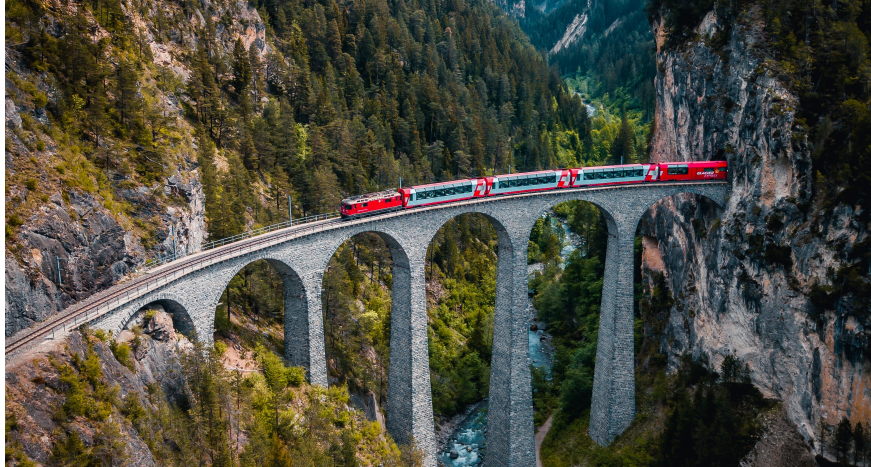
Fig. 7.12 Overhead line equipment installed on a line passing from a tunnel to an exposed environment on the Landwasser viaduct, Switzerland. Image from [311].
