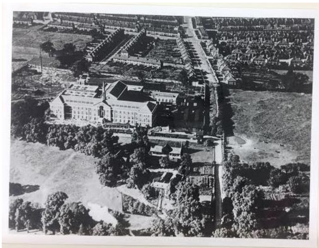
5.12—Aerial photograph of Research Station at Dollis Hill, c.1933/34 (PMA: POST 76/47). 77
