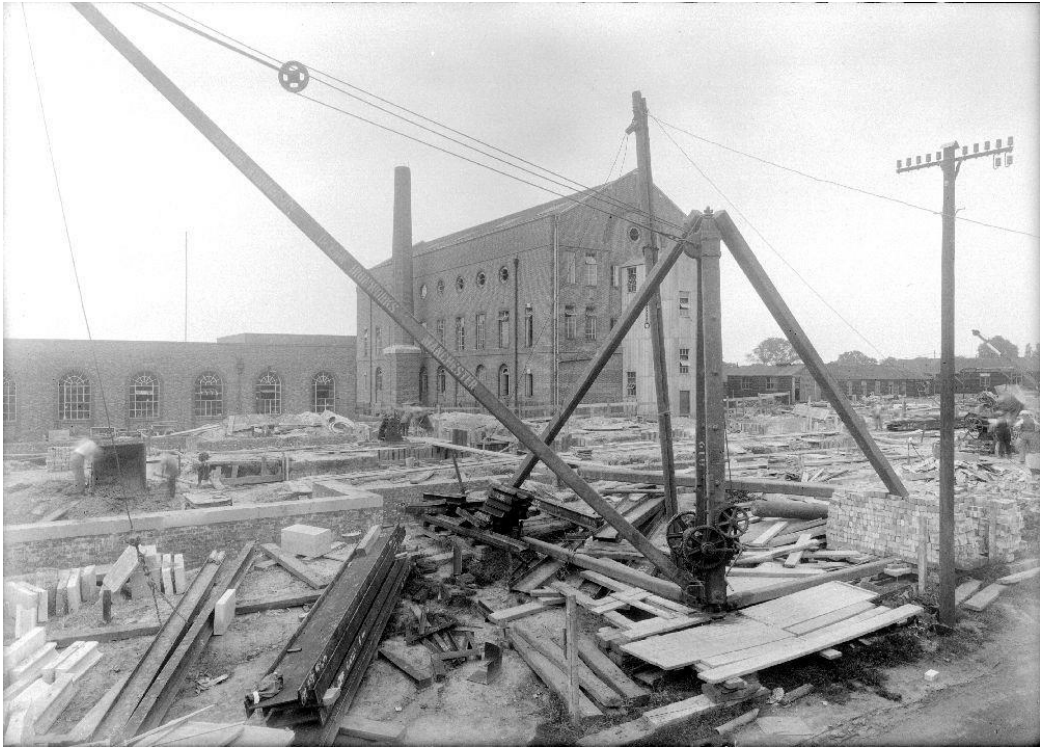
5.9—Construction of the permanent buildings, c.1931-32 (BTA: TCB 361/ARC 376).
