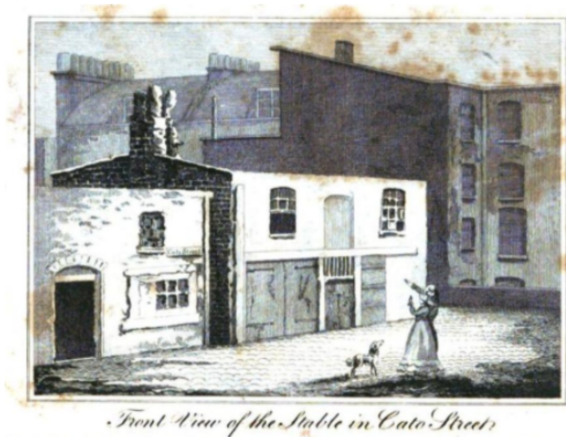
Front View of the Stable in Cato Street Figure 83: Front view of the stable in Cato Street (Aylmer 1820). This view places the stable into its landscape, demonstrating its ordinariness.
