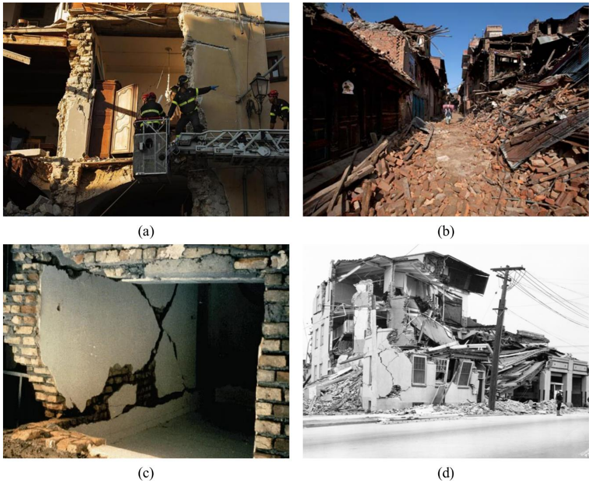
Fig. 1.1 URM failures during earthquake events: (a) L’Aquila, Italy, 2016 – Mw 6.3, (b) Kathmandu, Nepal, 2015 – Mw 7.8, (c) Rasht, Iran, 1990 – Mw 7.4 and (d) Long Beach, California, 1993 – Mw 6.3.
