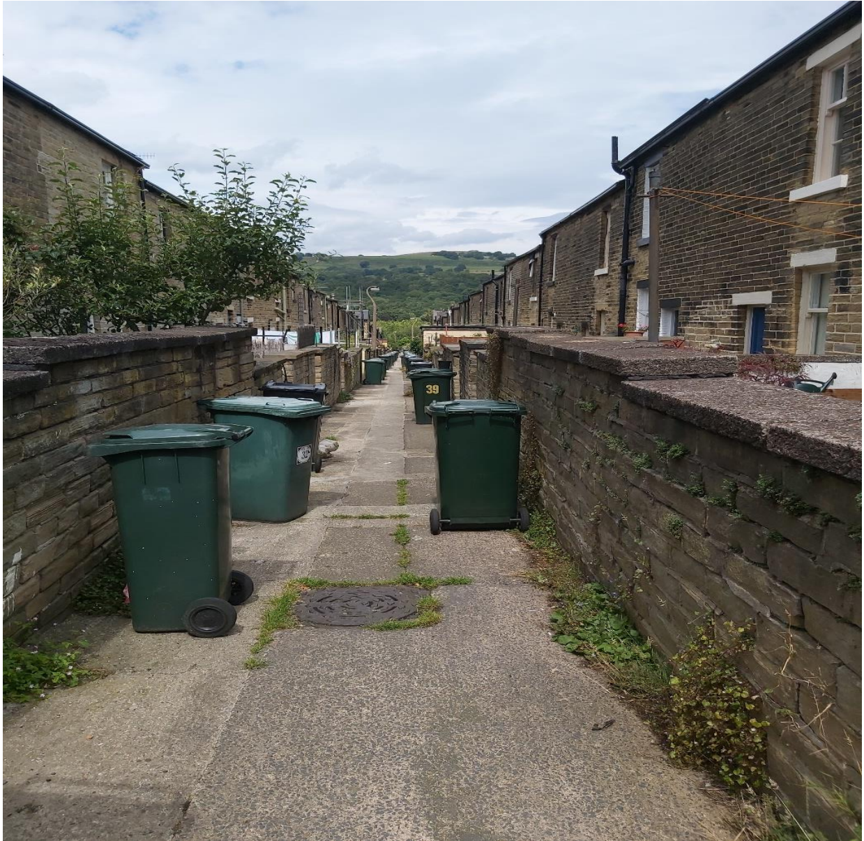
Figure 45. Writer's own photograph of back-to-back Saltaire Houses showing small yards and privvies taken, July, 2020.
