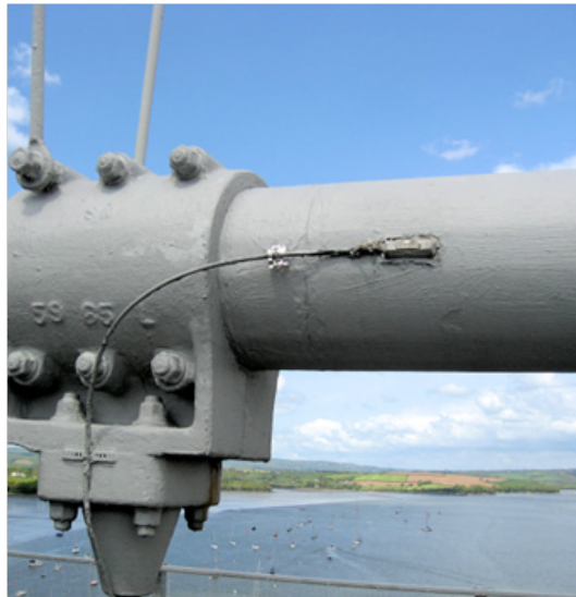
Figure 4.5: Thermogauge on the outside of the suspension cable.
