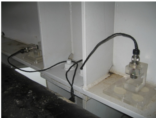
Figure 5.2: Accelerometers located on the truss.
