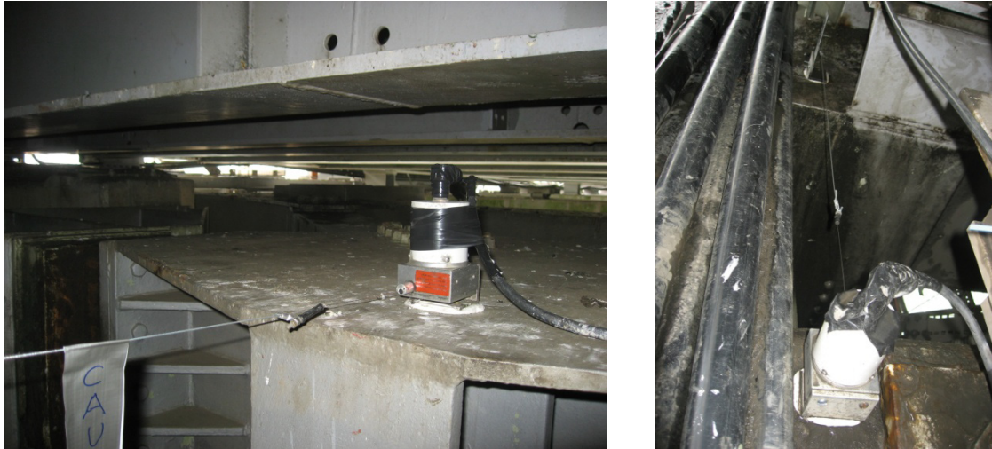
Figure 4.6: Extensometer mounted across the expansion joint.
