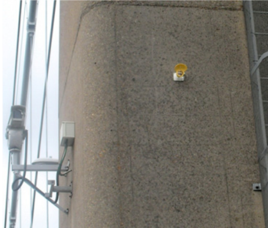
Figure 4.8: Reflector located on the side of a Saltash main tower.
