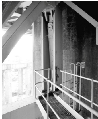
Figure 3.7: Rocker elements on towers.
