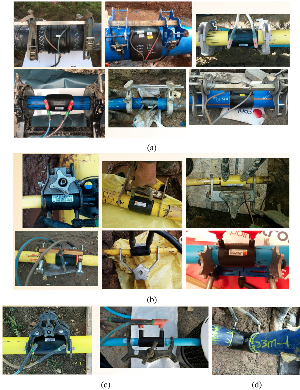
Fig. 4.1 Some examples of different styles of clamp in water and gas pipe images. (a) Ring clamps. (b) Metal pinch clamps. (c) Plastic pinch clamps. (d) No clamp.
