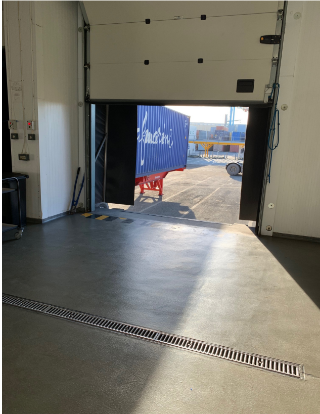
Figure 8. Showing part of the inspection area with containers parked up. Taken February 2019.
