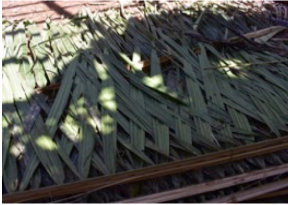
Picture 3 (left) shows the weaving technique using fresh tropical leaves to build the roofs of traditional Kichwa houses.
