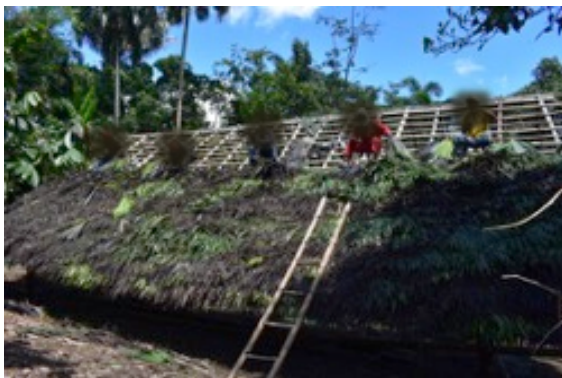
Picture 17 Men building the roof of a traditional house
