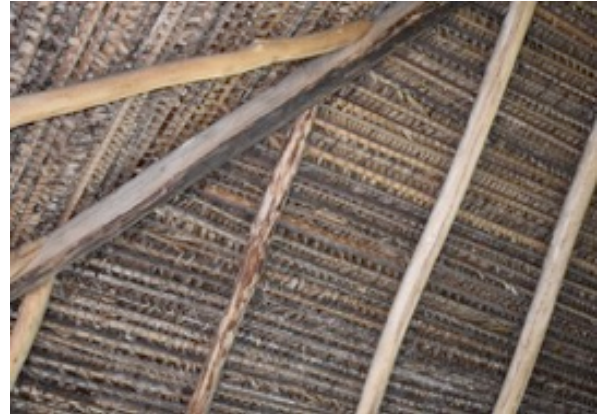
Picture 3 (left) shows the weaving technique using fresh tropical leaves to build the roofs of traditional Kichwa houses.
