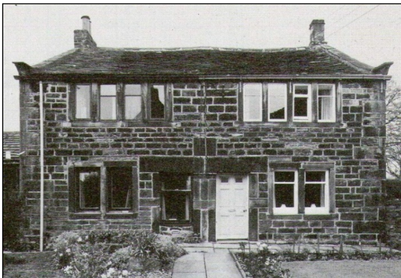
Nos 32 and 33 Oldfield. The large banks of windows on the upper floor are for lighting the weaving looms, set up above the living room and scullery on the ground floor. (Caffyn 1986, 11)
