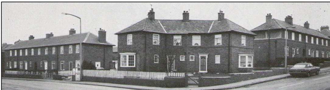
Figure 5-25: Estate for miners, Ryehill, Havercroft
