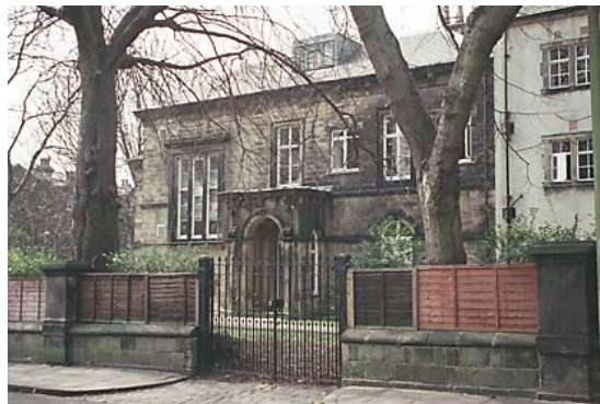
Mid 19 th century Regent Villas. Back-to-back semis associated with Devonshire Hall, University of Leeds. UID: 466229.
