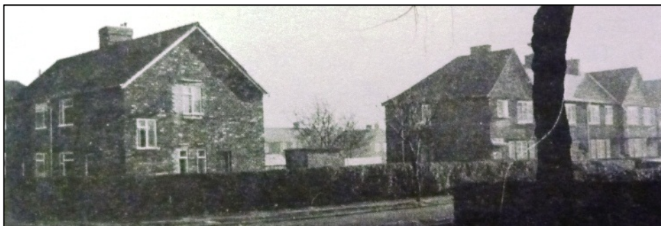
Non-parlour 1920 terraces (right) and the "infill" parlour semis (left) built in 1922 (Swenarton 1981, 183).
