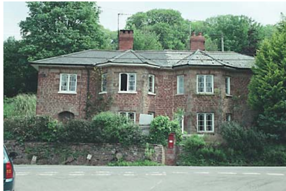
1824 Calverley Cottage, Woodford. Part of an emparkment village by Sir John Treveleyan opposite the entrance to Nettlecombe Court. UID: 264805.
