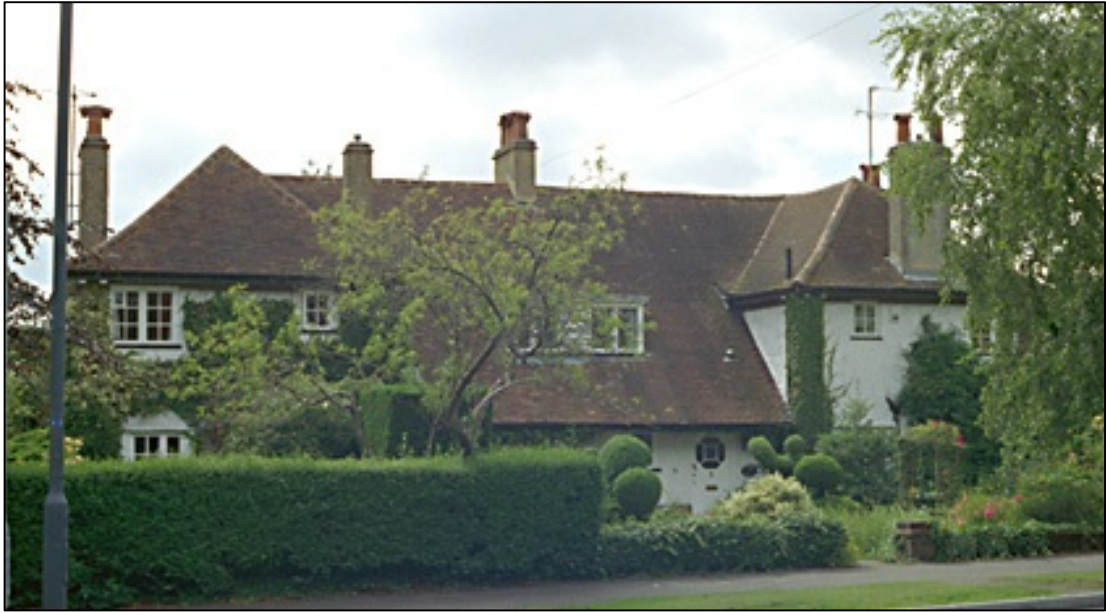
Nos 3 and 5 Norton Way North (English Heritage, Images of England, 161942)
