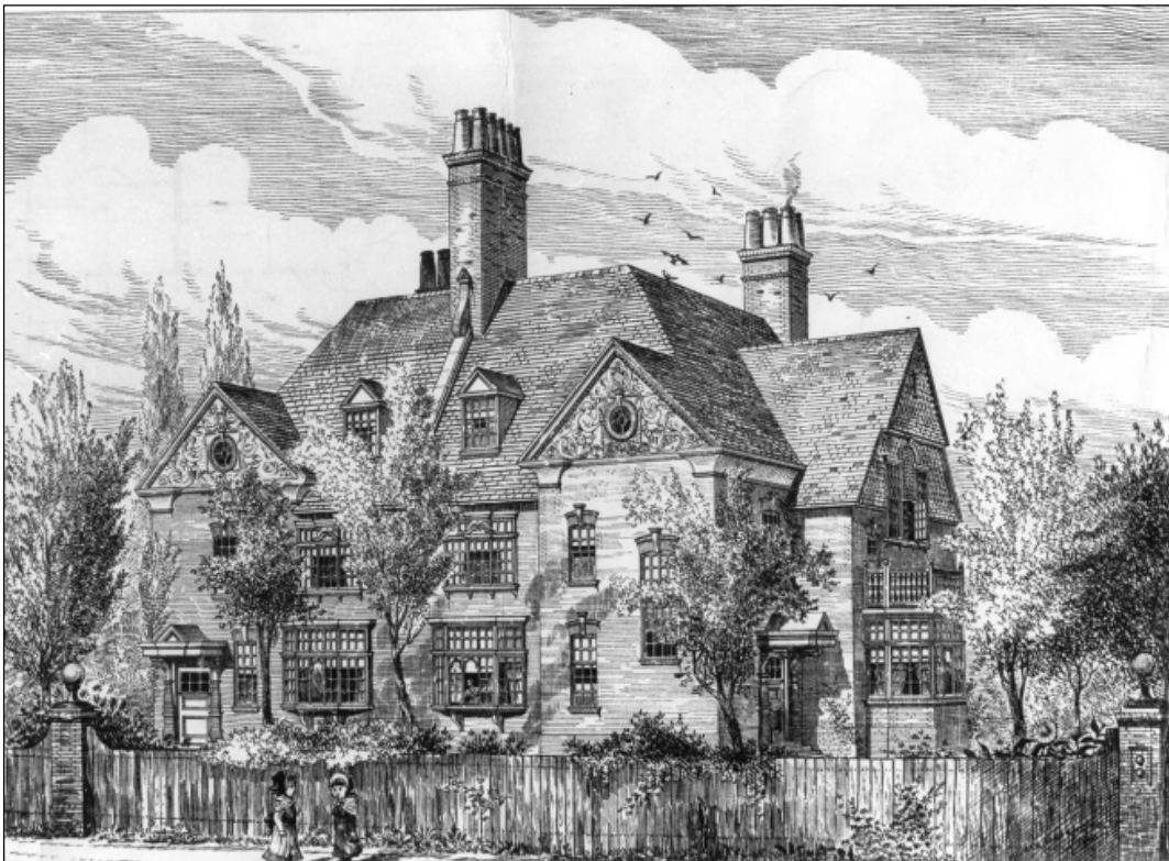
Semis designed by architect Maurice Adams at 12-14 Newton Grove. The entrances are designed to enhance the appearance of the semis as one large villa. (The Bedford Park Society www.bedfordpark.org , accessed 23 August 2011).
