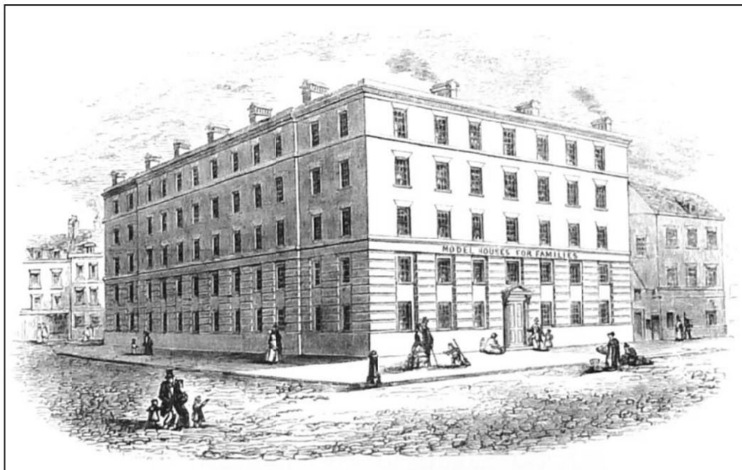
Model houses for families, in Streatham Street, Bloomsbury, built by the Society for Improving the Condition of the Labouring Classes (Roberts 1853, 49).
