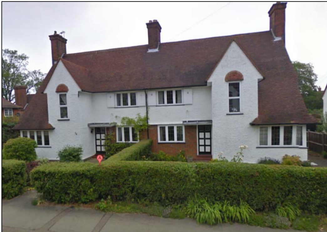
Nos 34 and 36 South View (Google Maps, accessed 6 January 2012)
