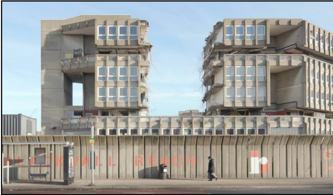
Figure 22: Demolition at Robin Hood Gardens begins, 2017 (Frearson 2017).
