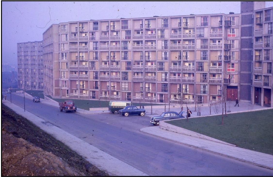
Figure 13: Park Hill flats on South Street in 1961, highlighting the gradient change in the brick infill panels (from Sheffield History 2020).
