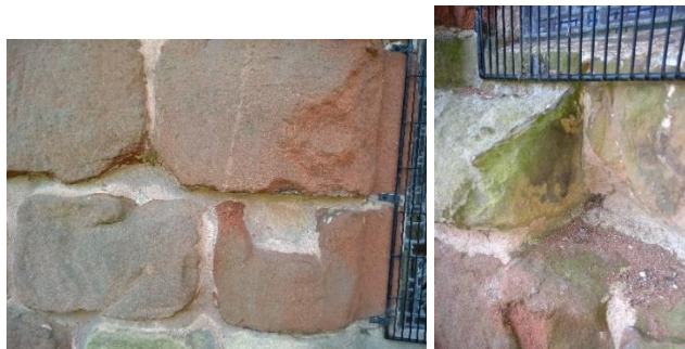
Fig. 3.28. Features mentioned by Cranage that he suggested may have been related to the building of an anchorite cell—but are really putlog holes or other evidence of later construction.
