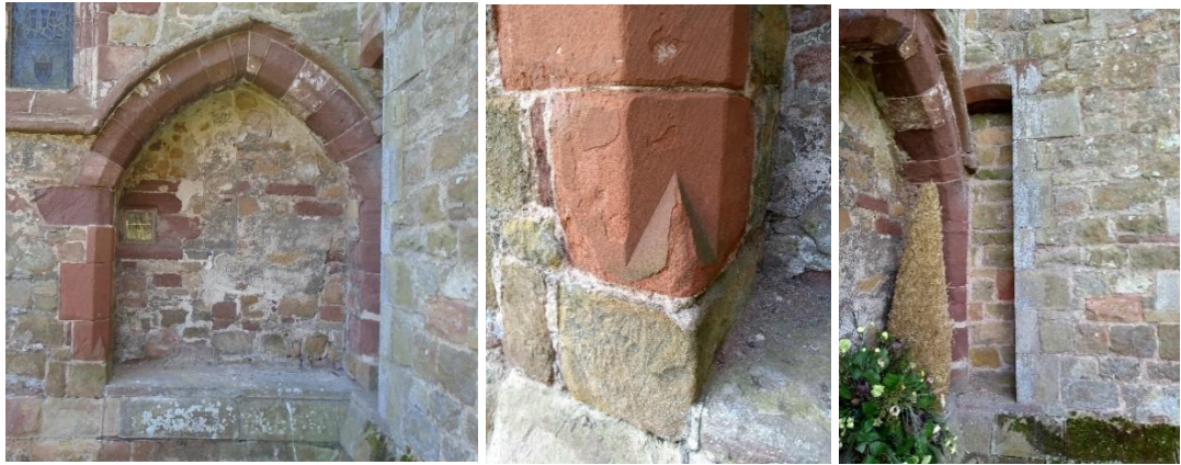
Fig. 3.13. The Acton Burnell arch, with the foundation creating a platform visible (left); an example of newer stonework added to the arch (middle); and the niche cut out of the tower to preserve the arch (right).
