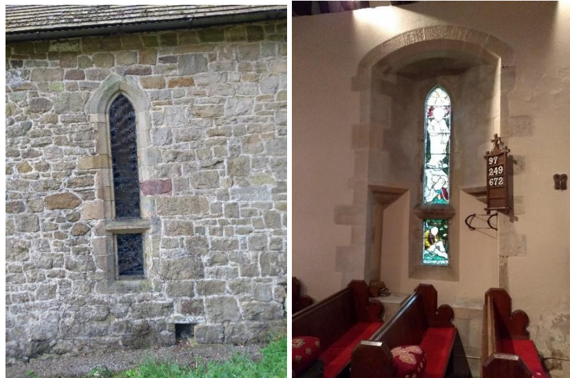
Fig. 3.46. An external view of the distinctive lancet window with the rectangular window below, very close to the squint (left); and an internal view of the same window, showing the niche it is placed in, distinct from other nave or chancel windows (right).
