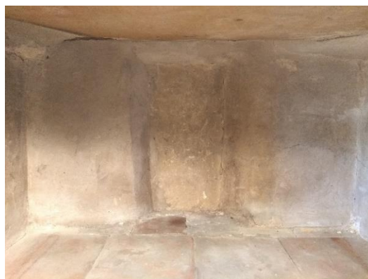
Fig. 3.4. The splayed squint-style window in the first storey of the eastern wall at Much Wenlock.
