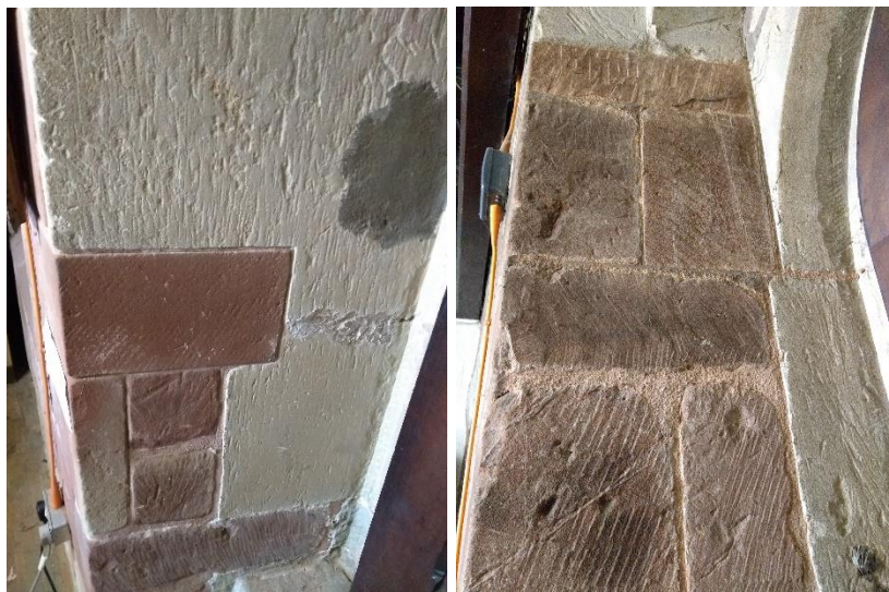
Fig. 3.36. Close-up views of the doorframe next to the squint recess, showing the continuation of the medieval build.
