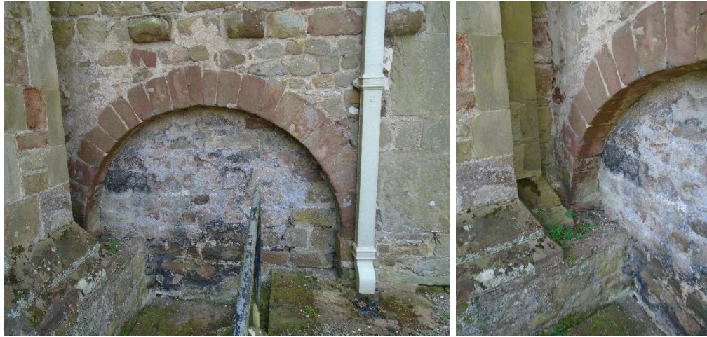
Fig. 3.16. The rounded arch at the end of the transept, below the corbel table. Note also that the raised foundation ends at this point.
