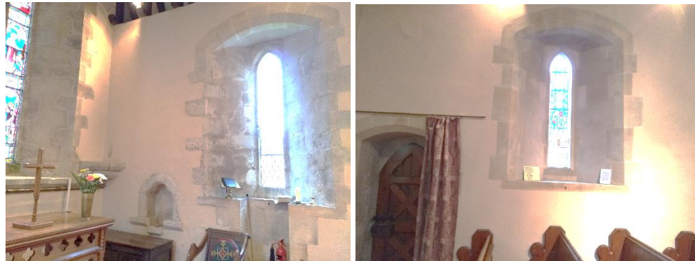
Fig. 3.57. The distinctive lancet window close to the altar (left), and a comparison to the lancet-style windows in the chancel and nave set into typical recesses (right).
