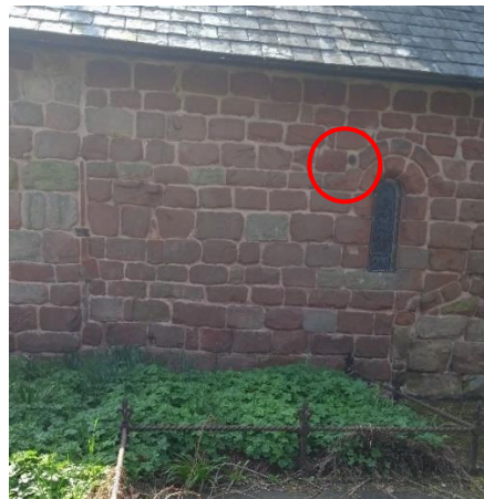
Fig. 3.27. Before the chancel extension was added, the continuous string coursing between the Norman windows stopped with a now worn circular decoration.
