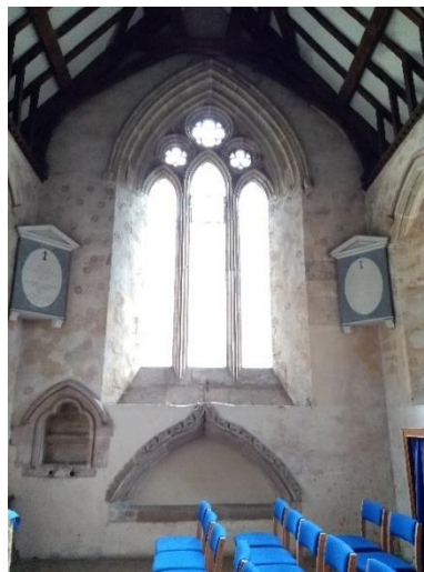
Fig. 3.20. A comparison view of the south transept—although the piscina and window have individual string coursing, the coursing does not link features and continue in a line around the transept.
