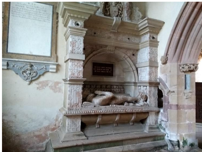
Fig. 3.17. The post-medieval tomb monument placed against the eastern wall of the northern transept. Note the partially covered piscina, and that the space where the arch now stands has been left blank, with plaster covering it.
