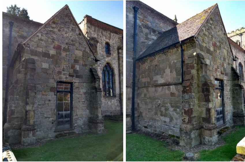
Fig. 3.40. The patchwork of phasing on the north wall of the cell, showing that the lower and upper parts of the north wall have been replaced with modern stonework (left); and the foundation ledge visible on the east wall of the cell (right).
