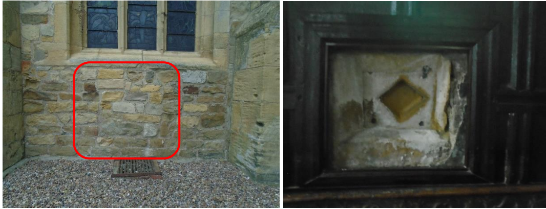
Fig. 3.31. The rectangular blocked squint recess at Barnburgh, Yorkshire (left), and the internal diamond-shaped squint placed within the recess, now surrounded by post-medieval panelling (right).
