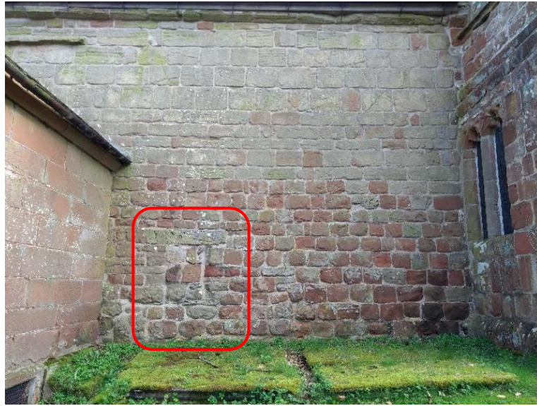
Fig. 3.29. The north chancel wall at Great Ness, with the blocked squint recess outlined in red. The modern schoolroom/vestry is in view next to the blocked recess.
