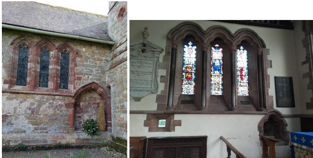
Fig. 3.19. The continuous external string coursing around the squint recess and windows (left); the continuous internal string coursing around the squint, windows, and piscina (right).
