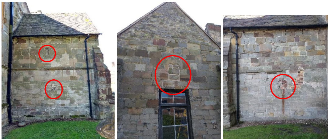
Fig. 3.11. The east (left), north (middle), and west (right) sides of the vestry, with the signs of windows circled in red.
