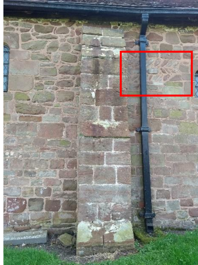
Fig. 3.42. The buttress blocking the location of where the medieval cell would have been placed. Note also the herringbone pattern next to the buttress.
