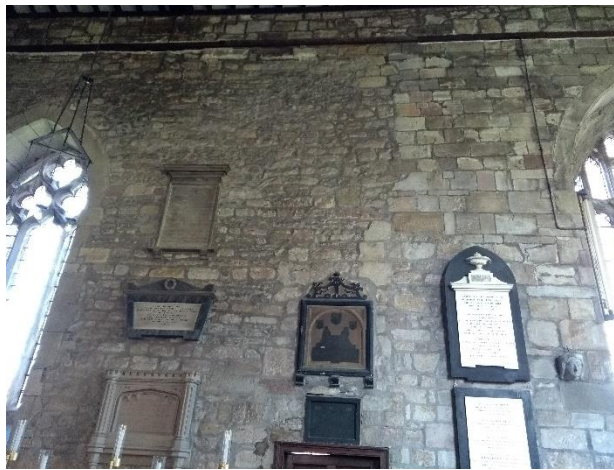
Fig. 3.41. The clear difference between the pre-chancel extension build, and the chancel extension stonework.
