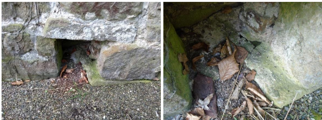
Fig. 3.44. A close-up of the lintel stone placed over the squint (left); and the rough internal walls of the squint, exacerbated by weathering (right).
