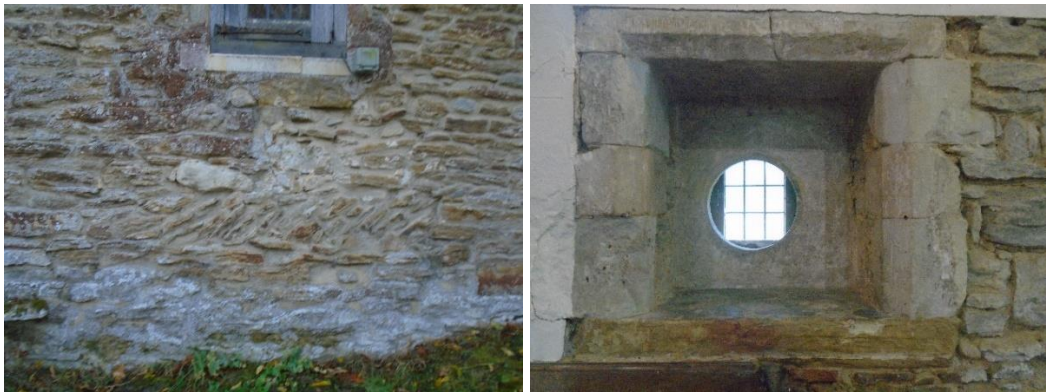
Fig. 3.53. An example of the herringbone stonework associated with the Staplehurst squint, directly underneath the squint (left); and an internal view of the large square squint (right). The niche cannot be seen because of the post-medieval addition of the masonry with the circular hole, designed to accommodate a flue.
