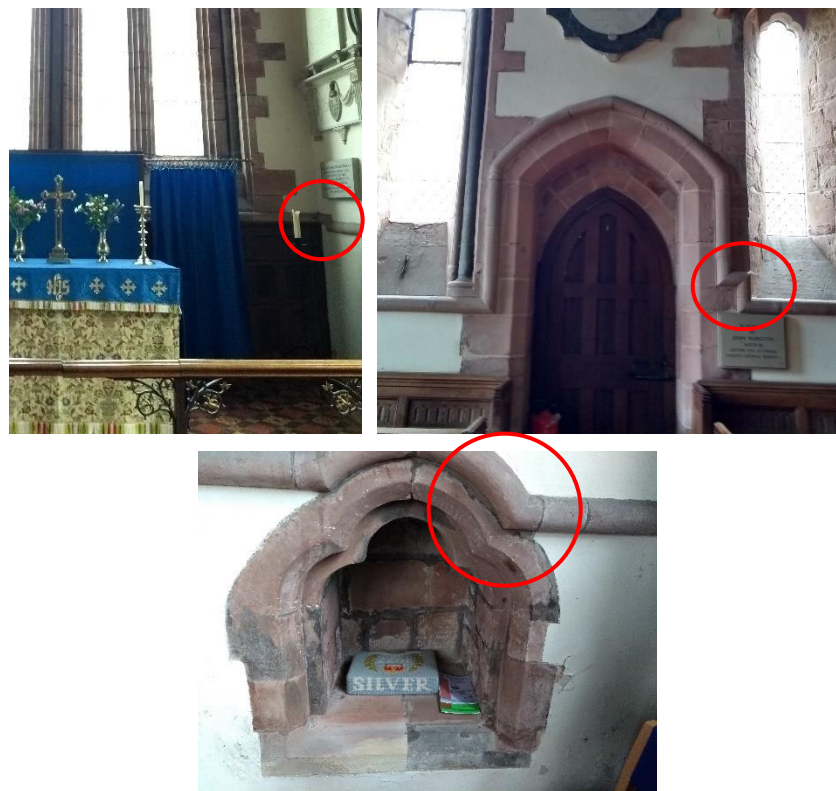
Fig. 3.21. Examples of the irregular continuous string coursing in the chancel at Acton Burnell, circled in red.
