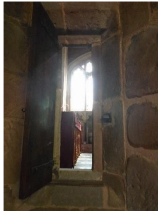
Fig. 3.2. The rebate for the wooden shutter, integrated into the medieval build.
