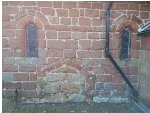
Fig. 3.23. The blocked squint recess at Ruyton, set between two Norman windows.
