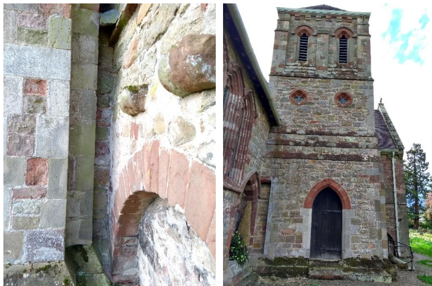
Fig. 3.15. A close-up of the corbel table and a gap between the post-medieval tower and the medieval transept (left); a view of the post-1888 tower—note that the design of the door arch complements the squint recess (right).
