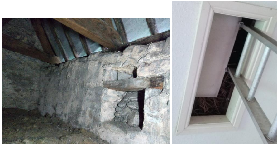
Fig. 3.7. One of the blocked squint-style window recesses in the second storey (left), and a view of the sliding panel allowing access to the second-storey, with a massive bird's nest blocking the entrance just visible (right).
