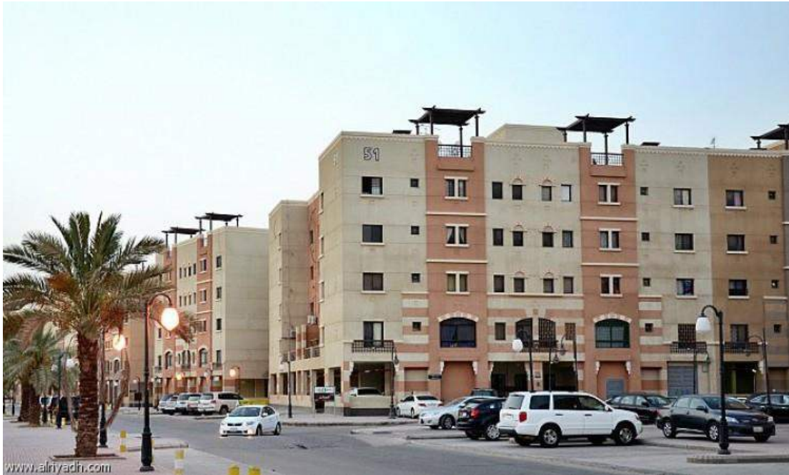
Figure 4.12: Apartment building in Riyadh, Saudi Arabia (Al-Riyadh, 2014)
