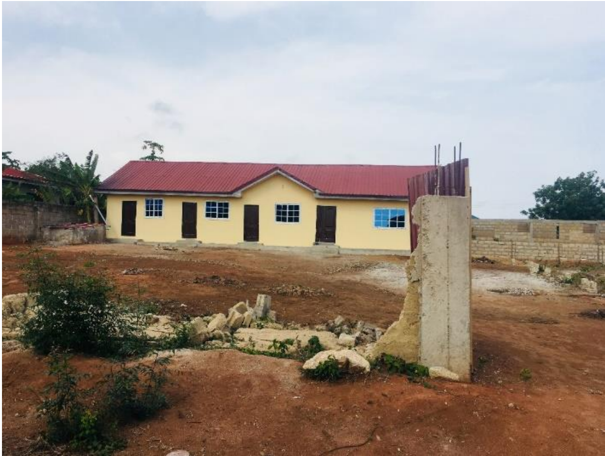
Plate 7.2. A fence wall demolished in Abokobi
