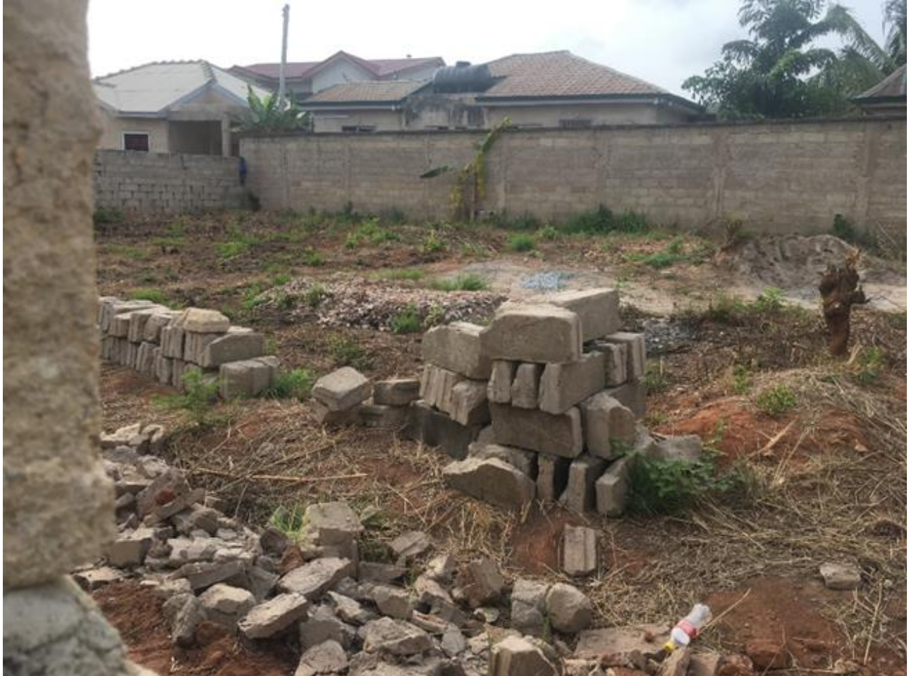
Plate 7.5. A wall built around a parcel of land as a form of protection
